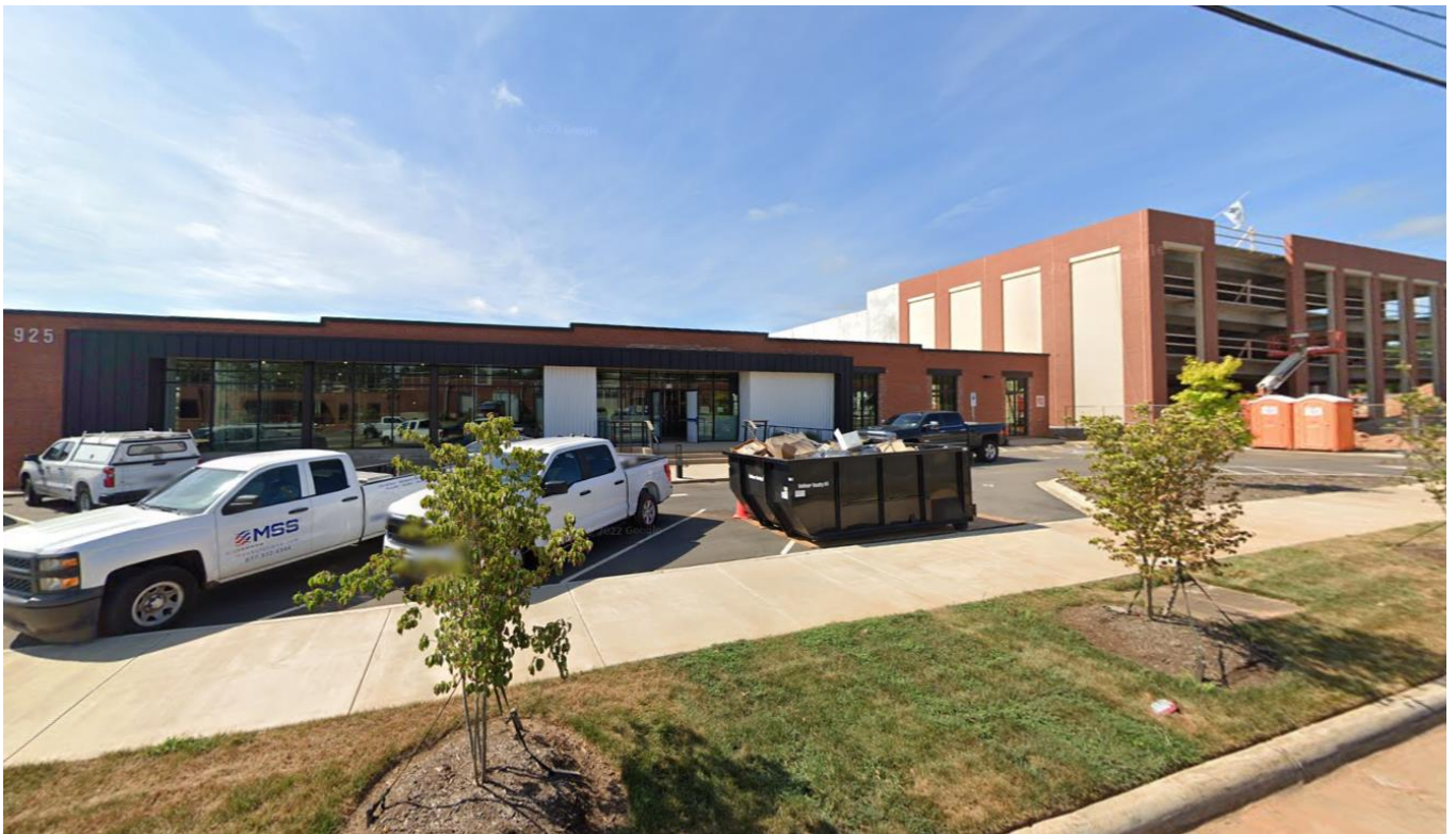
View of a completed adaptive reuse office project and another adaptive reuse project under construction located directly west of the site on Tuckaseegee Road.
