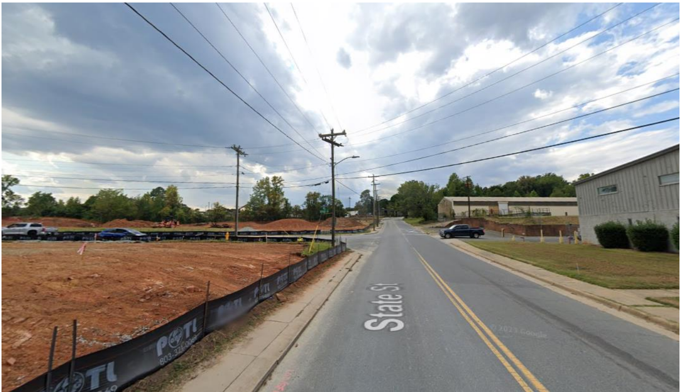
View of the intersection of State Street and Gesco Street, located north of the site. At the right of the image are active warehouses and at the left of the image is a site under construction that will contain mix of multi-family dwellings, single-family attached dwellings, and commercial uses.
