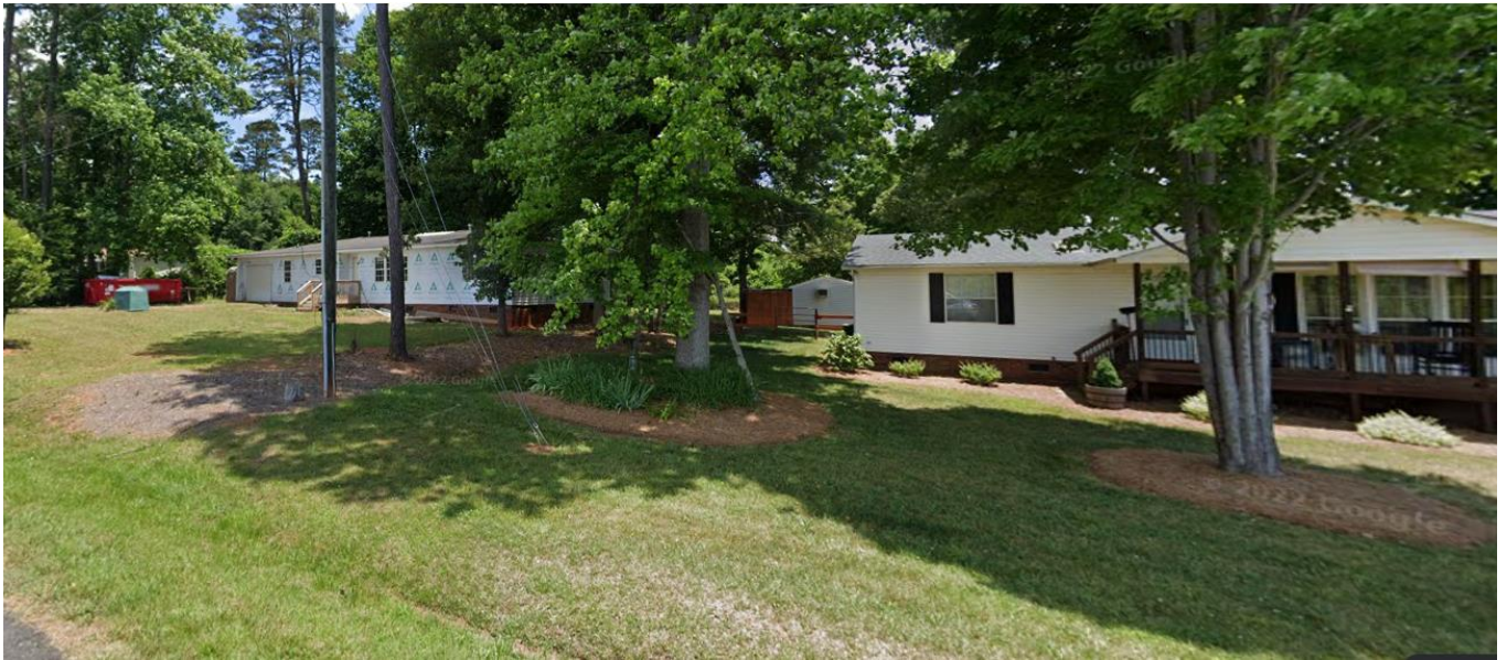
East are single family homes.
