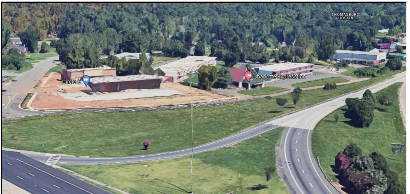
The property to the south is developed with a Circle K along Lucky Penny Street.
