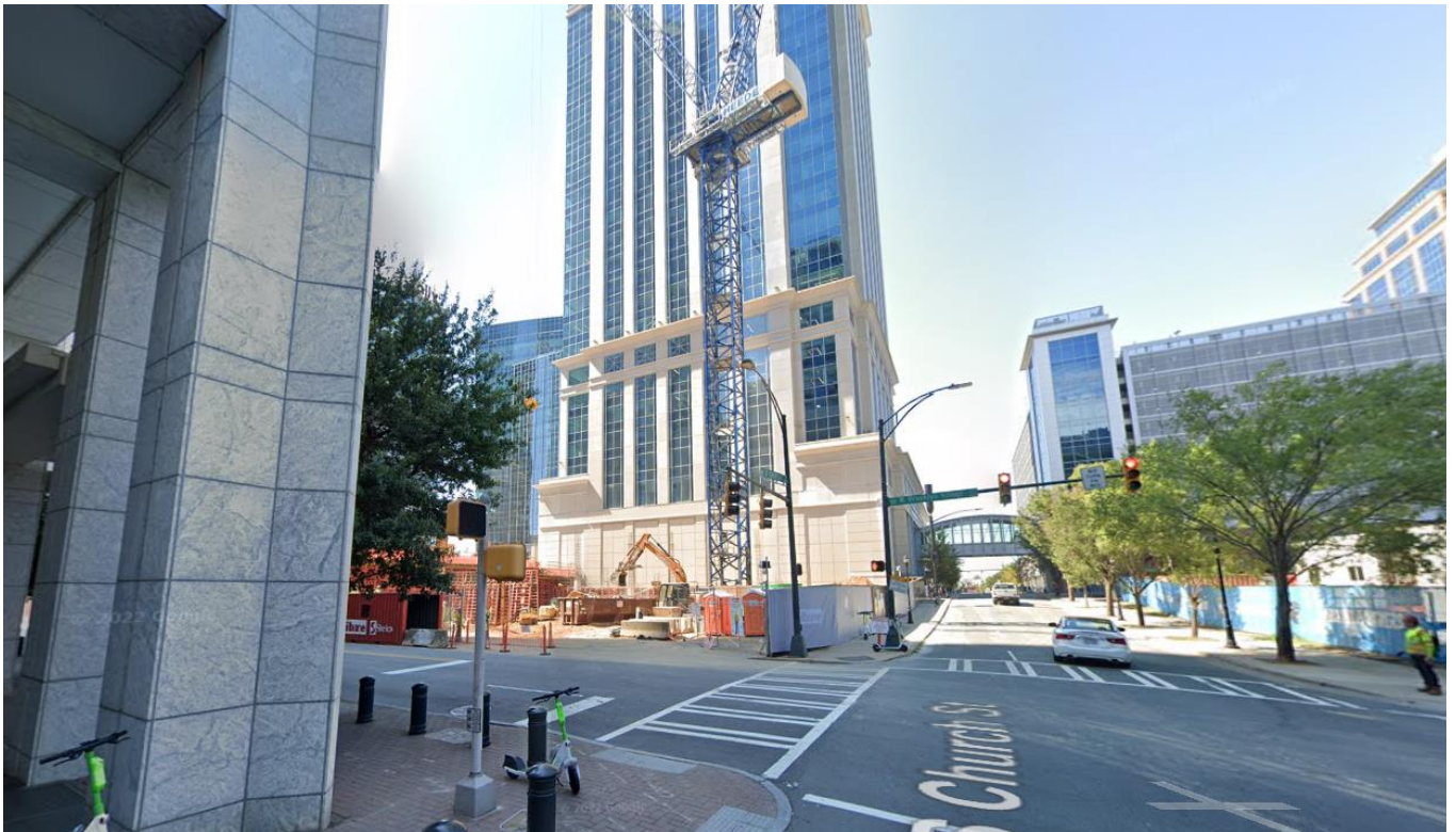
View of the site looking south from the intersection of South Church Street and East Brooklyn Village Avenue. The sign is proposed to be located on the building under construction at the southeast corner of this intersection.
