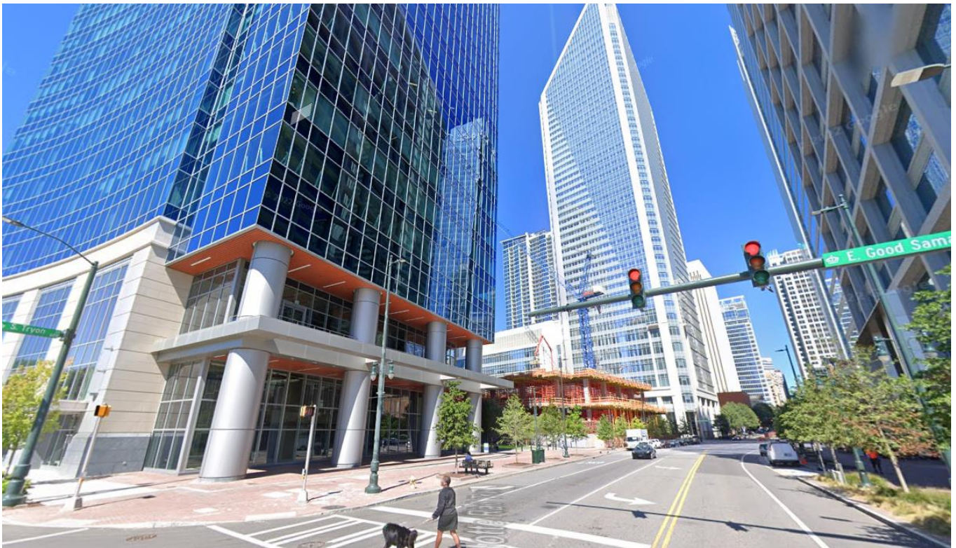
View of the site looking north from the intersection of South Tryon Street and East Good Samaritan Way. The subject building is under construction in this image and the Tryon Street plaza is located between the building on the left in the foreground and the building under construction in the bottom center of the image.
