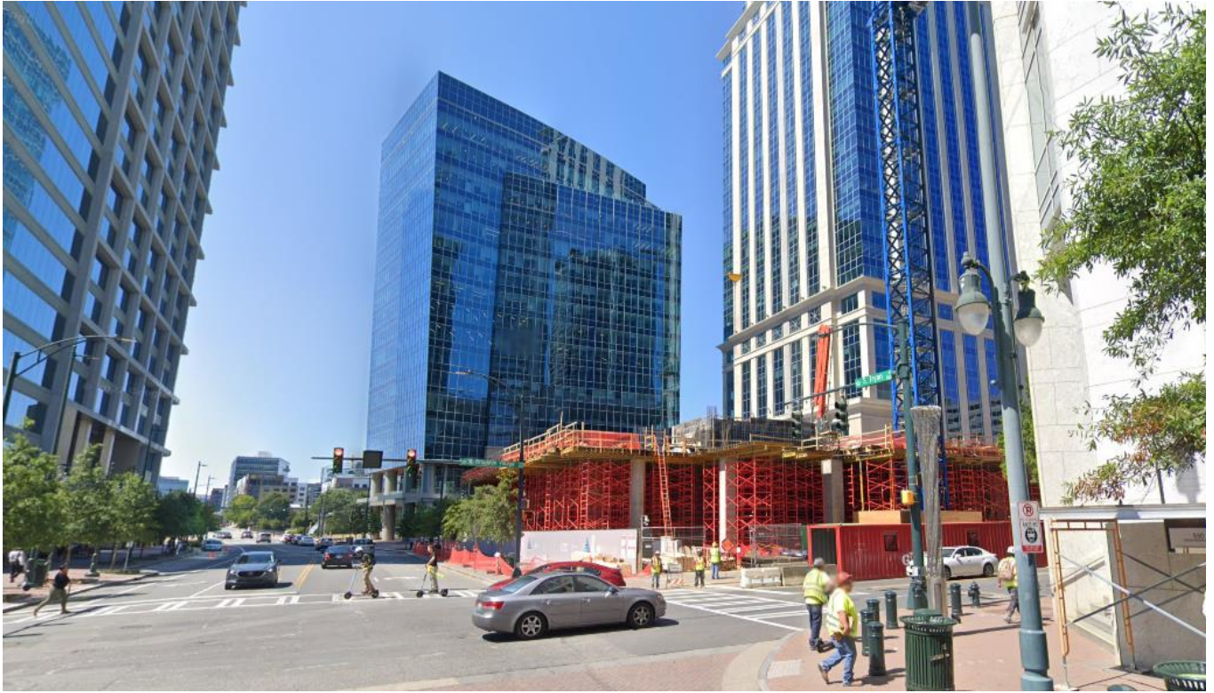
View of the site looking south from the intersection of South Tryon Street and East Brooklyn Village Avenue. The sign is proposed to be located on the building under construction at the southwest corner of this intersection.
