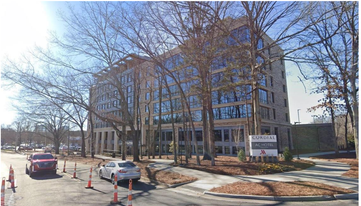
View of the AC Hotel located west of the site Across Roxborough Road.
