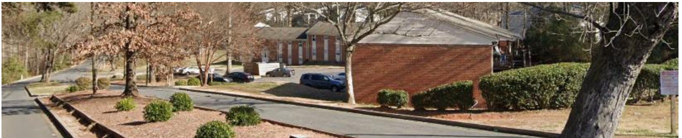
The property to the south of the site is developed with multifamily residential use.
