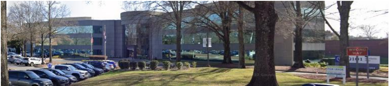
Streetview of office use to the east of the site across Southern Pine Boulevard.
