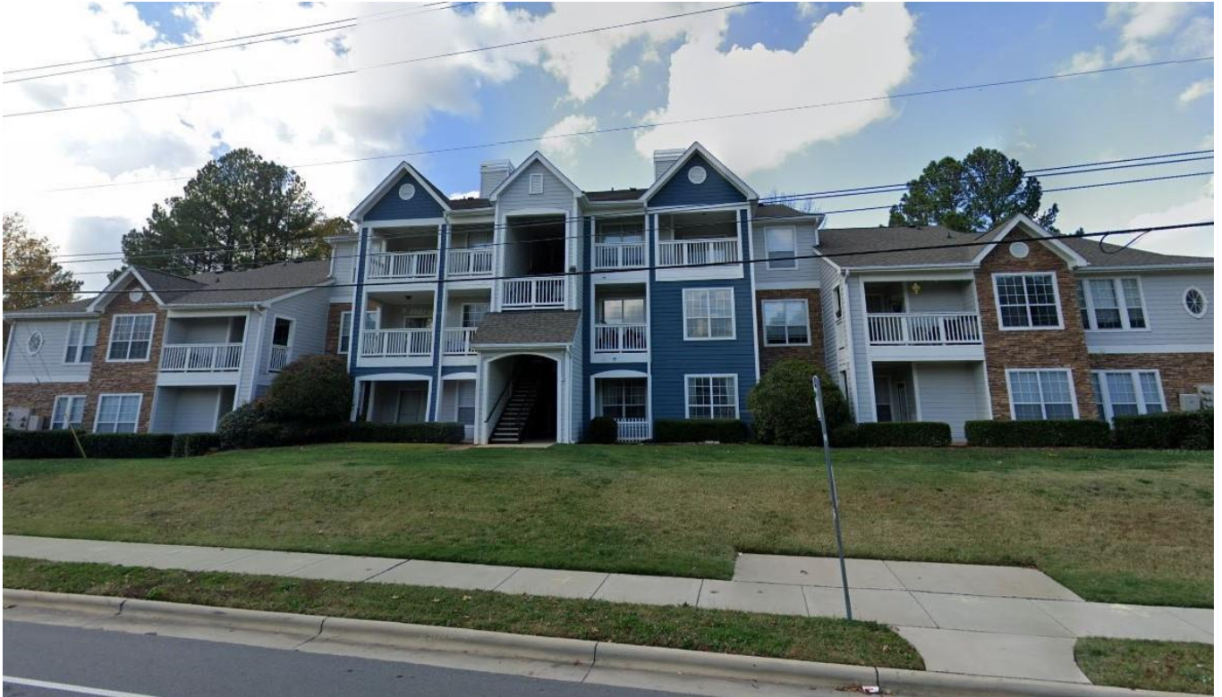
View of a multi-family development from Mallard Creek Road located to the west of the site.
