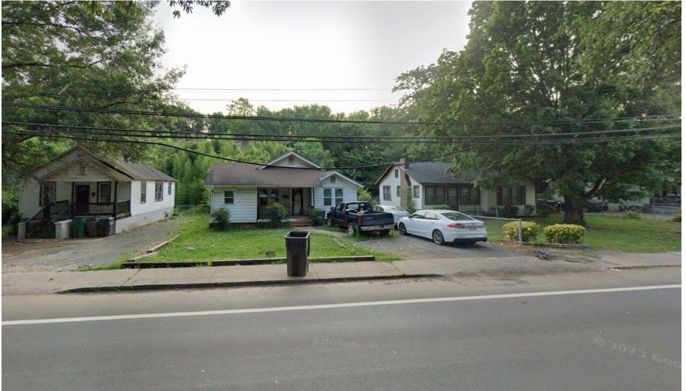
View of single-family homes located along Ashely Road zoned N2-B (neighborhood 2).
