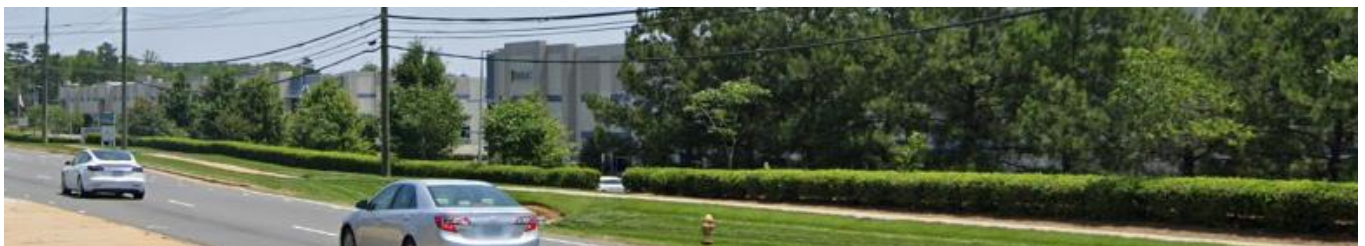
The properties to the east of the site across Steele Creek Rd are developed with industrial uses.
