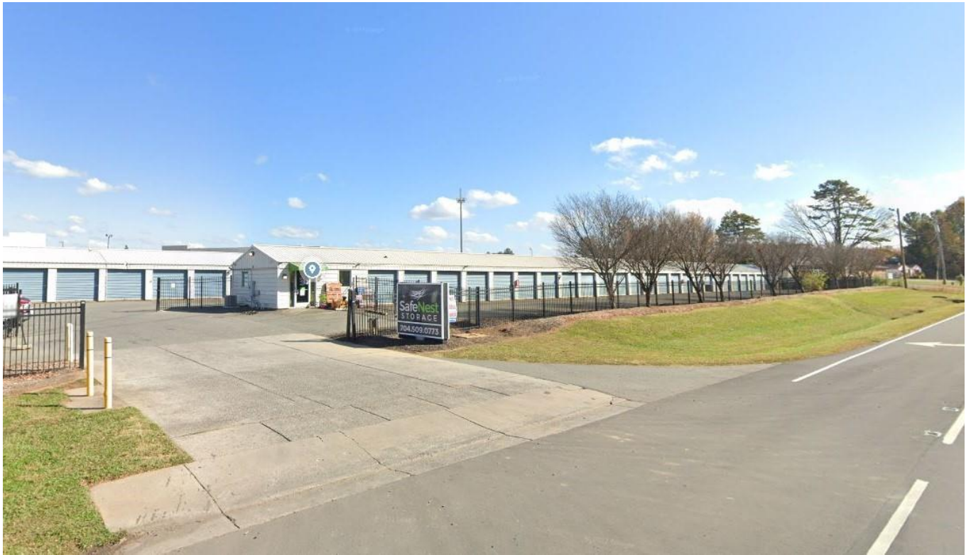
View of the site looking east from the Statesville Road. The property is currently developed with a self-storage facility.
