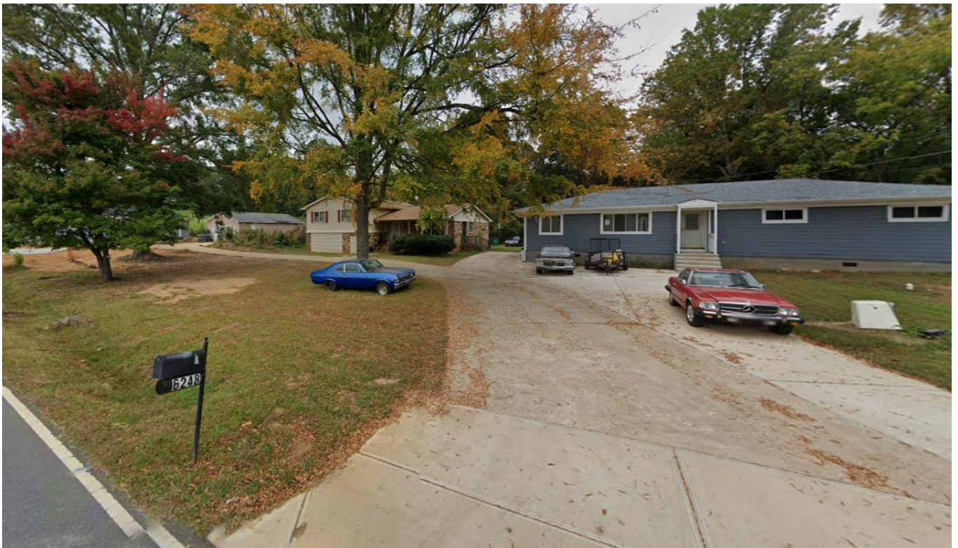
View of single-family houses located along Paw Creek Road, southeast of the site.
