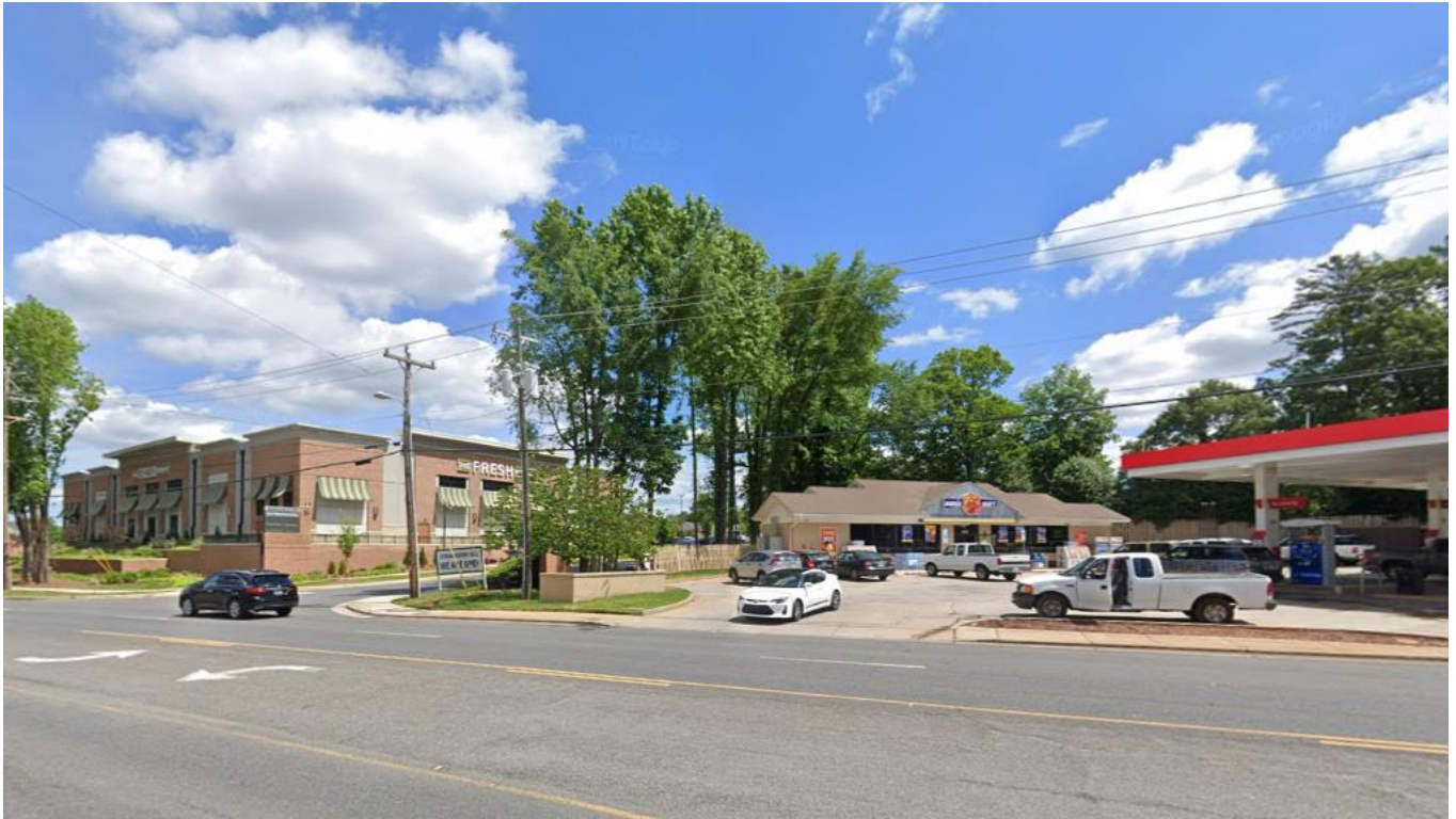
View of the Strawberry Hill development located at the north corner of the Providence Road and Sardis Road intersection located across providence Road from the site. Strawberry Hill is a mixed-use development containing retail, restaurant, institutional, residential uses.
