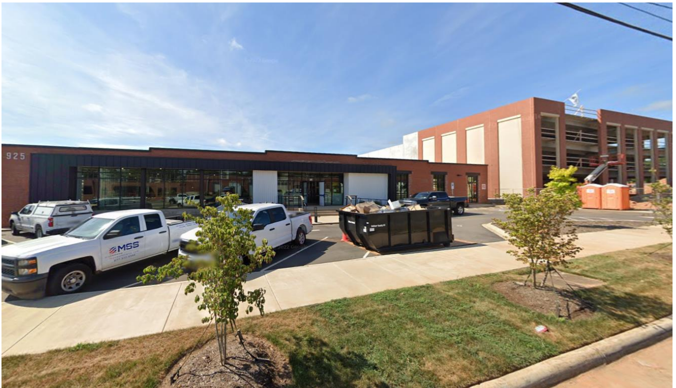
View of a completed adaptive reuse office project and another adaptive reuse project under construction located directly west of the site on Tuckaseegee Road.
