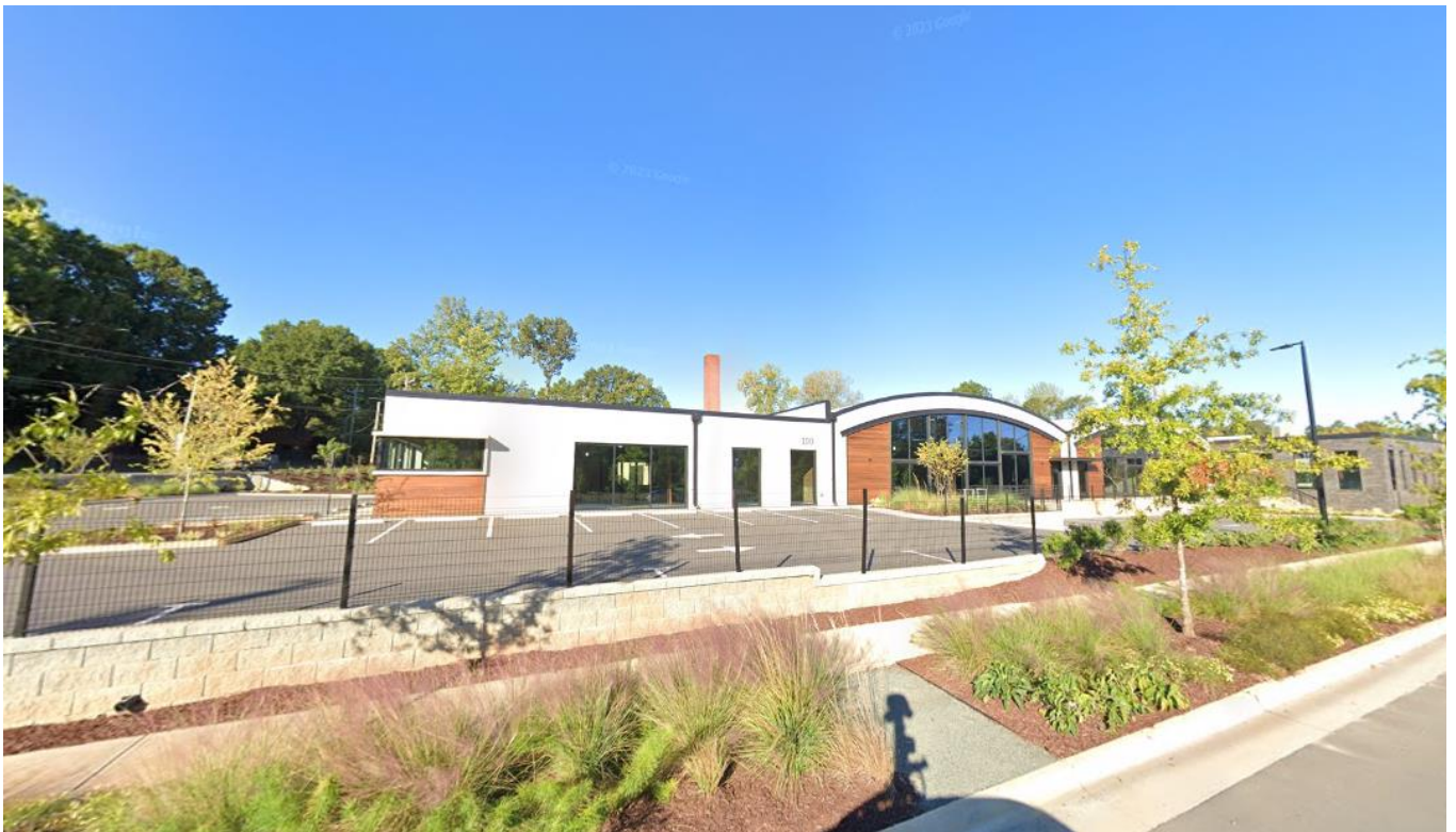
View of an adaptive reuse office project from the corner of Gesco Street and Tuckaseegee Road located directly east of the site.
