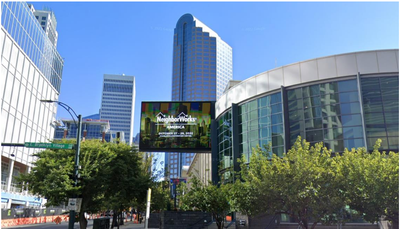
View of the electronic changeable copy projecting sign located on the Charlotte Convention Center. This sign is approximately 650 square feet per face and was approved by rezoning petition 2011-055.
