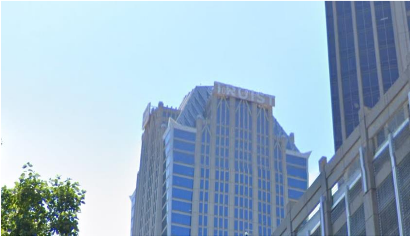
View of the Truist building skyline signs looking east from the intersection of West 6 th Street and North Church Street. The rectangular "Truist" sign is approximately 980 square feet. The square Truist logo sign located on the left side of the building in the image is approximately 558 square feet. The skyline signage was approved by rezoning petition 2020-064.
