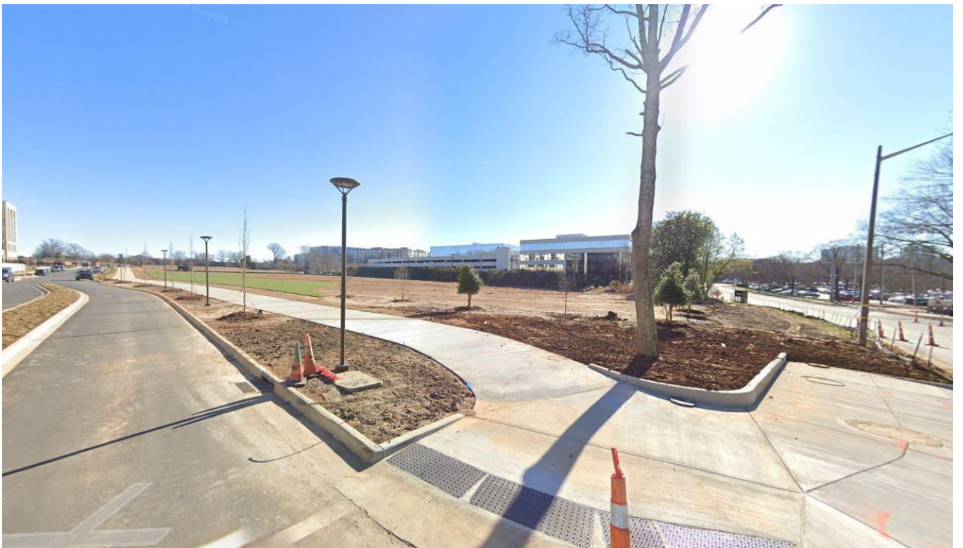
View of the site looking southeast from the intersection of Roxborough Road and Roxborough Parkway.
