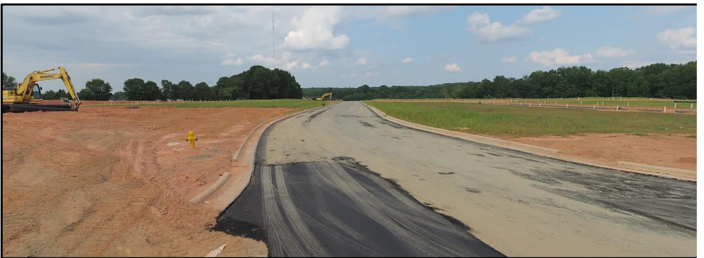
The property to the east along Bailey Run Drive is under construction for a townhome community.
