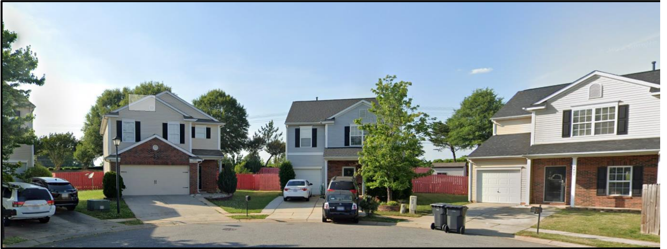
The property to the south across Rocky River Road is developed with single family homes.
