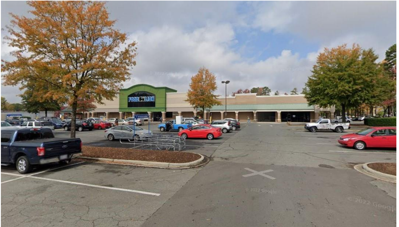
View of the Food Lion shopping center located at the northwest corner of Alleghany Street and Ashley Road within a ¼-mile walking distance of the site. There are several retail developments located within 1-mile of the site.
