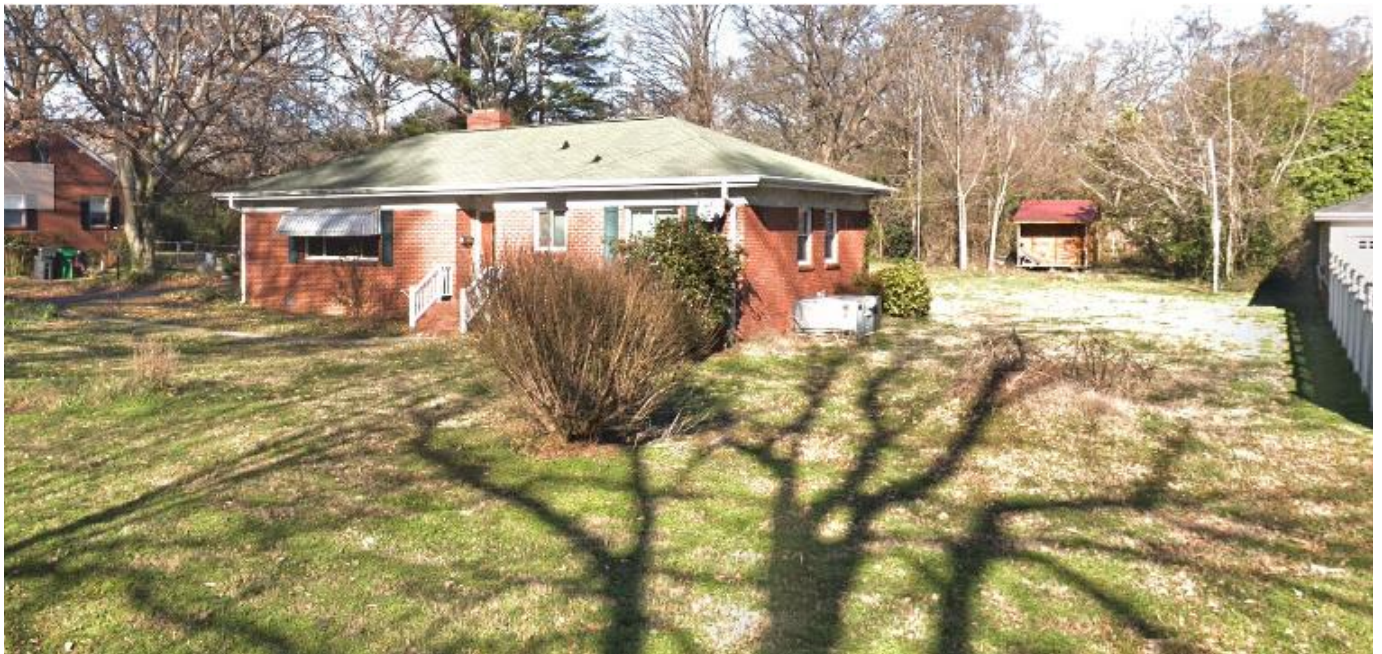
The site is developed with a single-family residential home constructed in 1952.
