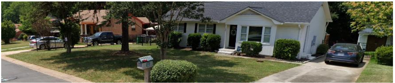
The properties to the south of the site are developed with single family residential use.
