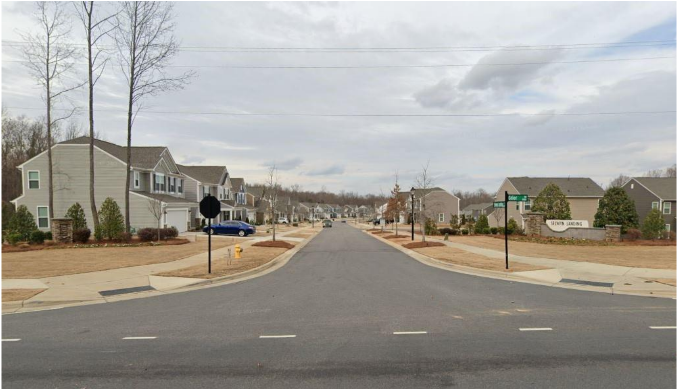
View of the Selwyn Landing subdivision located to the east of the site across East WT Harris Blvd.
