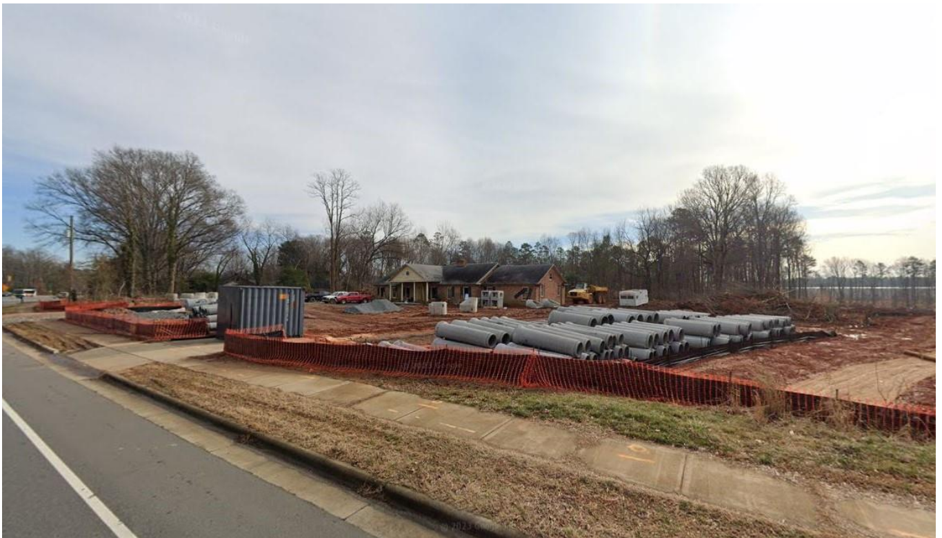
View of a townhome development under construction to the north of the site along Mallard Creek Road.
