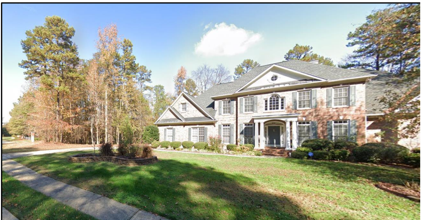
The property to the south along Lexington Approach Drive is developed with single-family homes.
