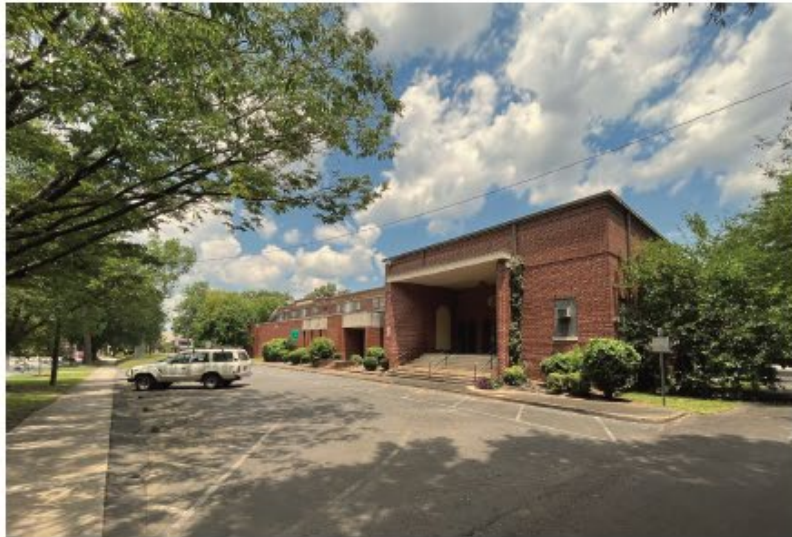
West Blvd, East side view of Wilmore School
