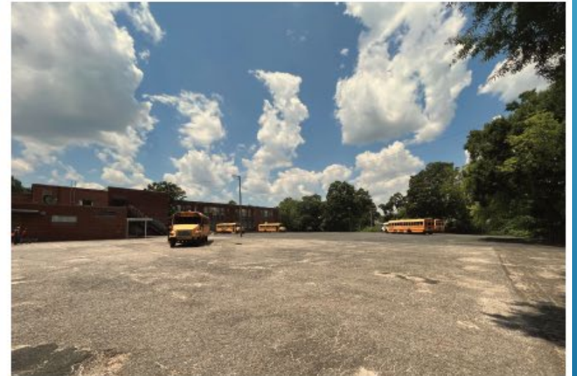
Rear Parking lot View, Wilmore School
