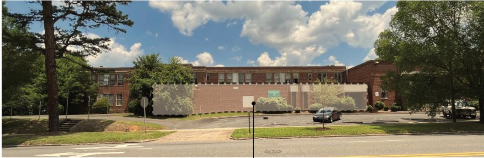
West Blvd, Front elevation of Wilmore School
