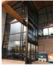
RAMM BK ALLUMINUM AND GLASS TUBE FRONT AND CURTAIN WALL 9 6 1/2 M BLACK ANODIZED AND CLEAR LOW E GLAZING
