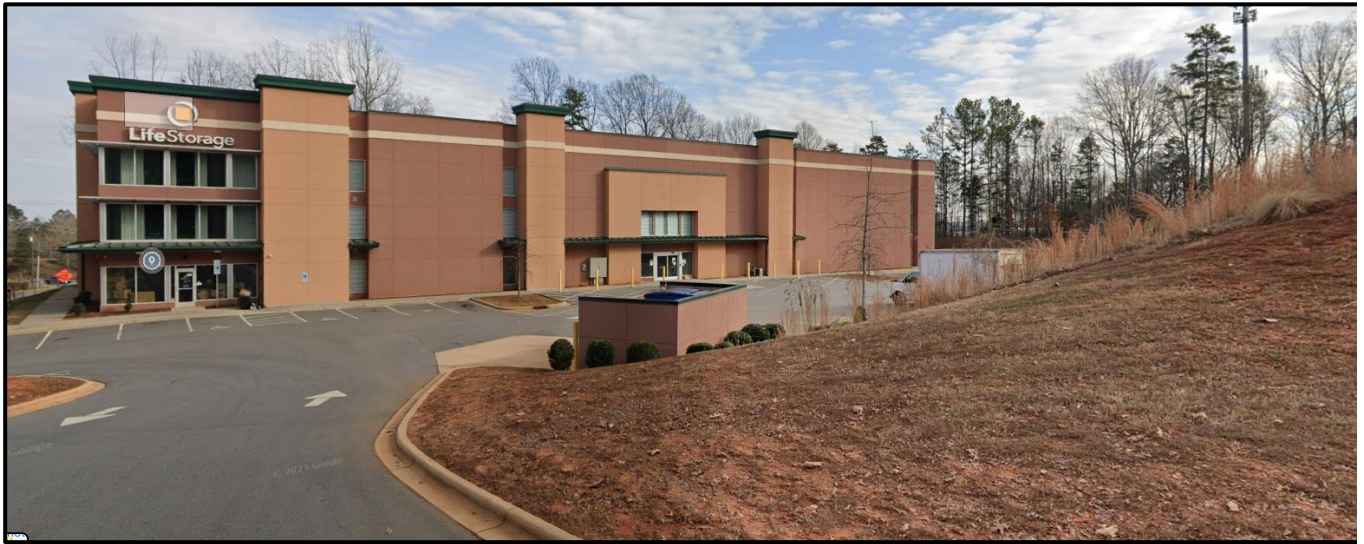
The property to the north along Legranger road is developed with a storage facility and a Duke Energy substation.
