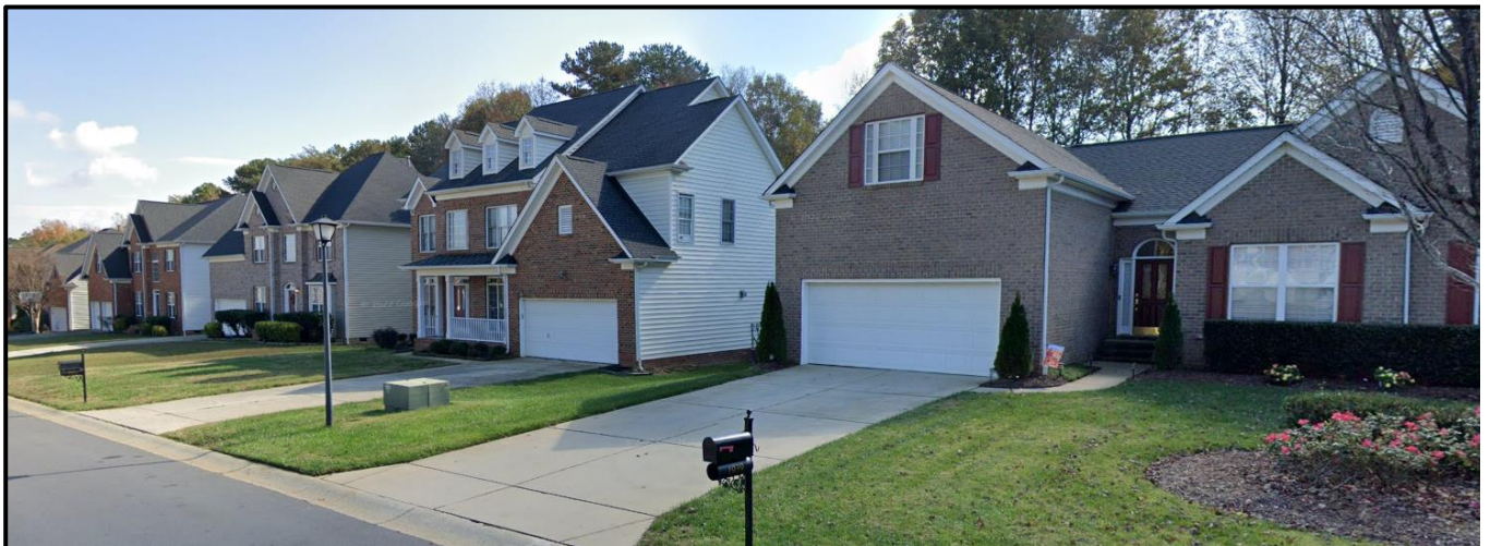
The property to the north along Copperplate Road is developed with single family homes.
