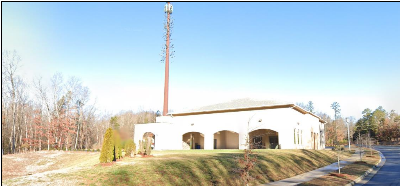
The adjacent property along John Adams Road is an event center and communications tower.
