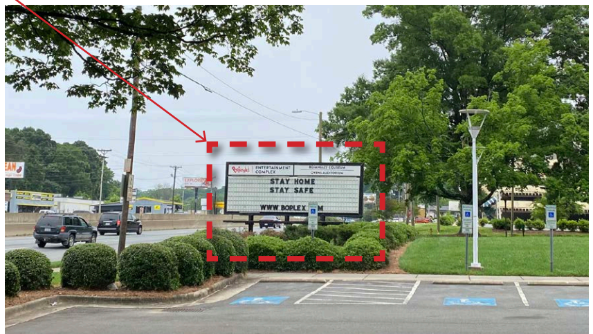
EXISTING MONUMENT SIGN TO BE REPLACED IN THE SAME LOCATION
