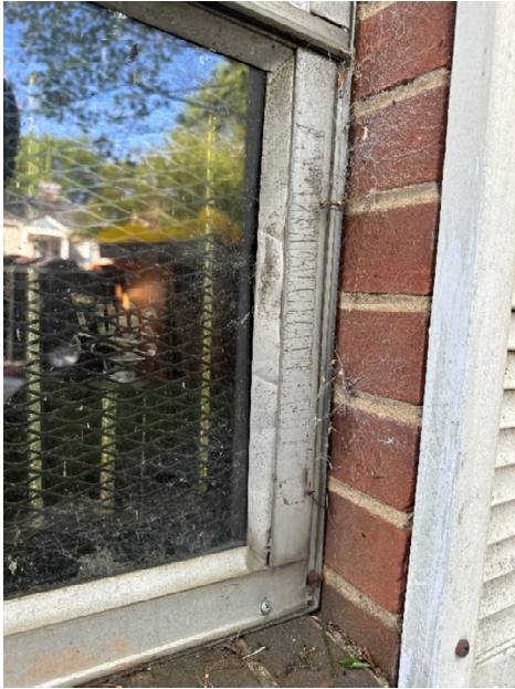
Exterior frame showing aluminum fatigue and self-taping screws installed through thermal envelope.
