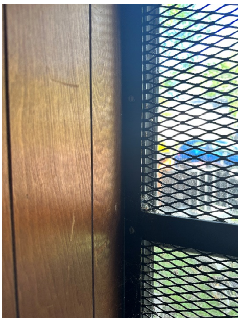
Interior: Self-taping screws used to affix mesh drilled directly into frame breaking the thermal envelope.
