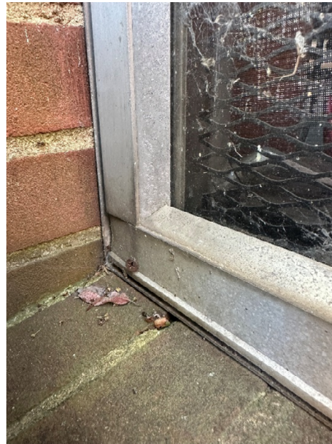
Exterior frame showing aluminum fatigue and self-taping screws installed through thermal envelope.
