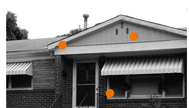
Wood is used for the trim surrounds, columns, eaves, railings, and brackets of the Bungalow above left while the Mid-Century Modern example uses wood only on the windows and trim, eaves and gable elements.
