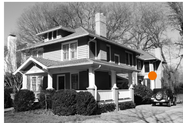
This two-story rear addition, like the example above, respects the vocabulary of the original dwelling with its hip roof, window proportions, and cladding.
