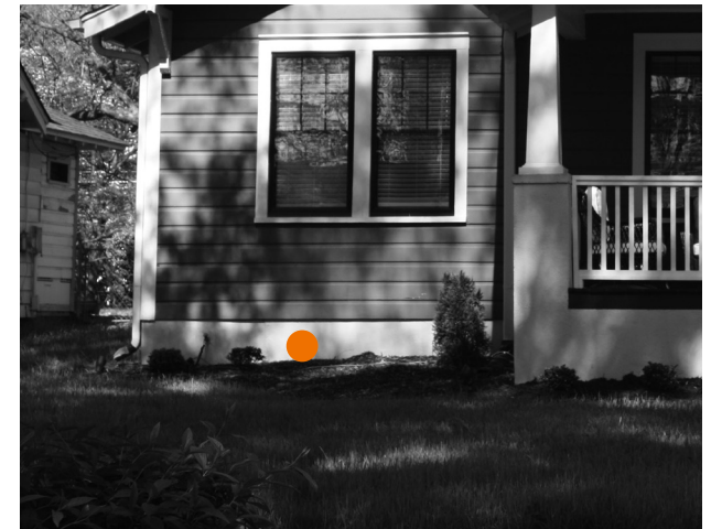
Stucco, like brick, provides a contrasting foundation material on this example.
