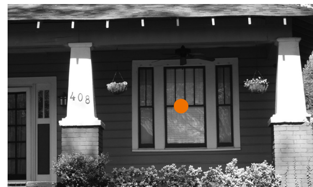
Bungalows with the Craftsman style influence usually have multi-light over single light windows such as the two examples above of three-part composite windows.
