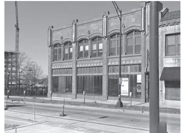
While this historic facade in Forth Ward retains a majority of historic features, the storefront has been modified by removing the entry door, however, original transom windows and display windows remain.
