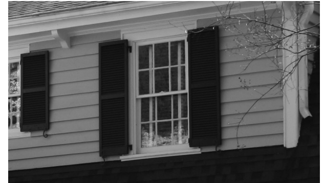
These shutters are properly sized for the window and hung on hinges. When closed the shutters fit the window opening.
