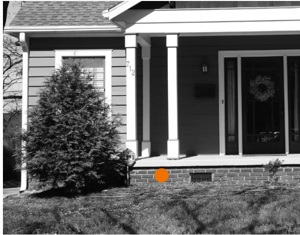
Brick is commonly found as a foundation material on many of the houses in all of the districts.
