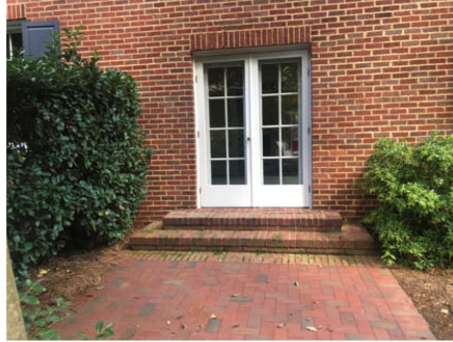
Existing Steps and Brick Paver at front south Terrace
