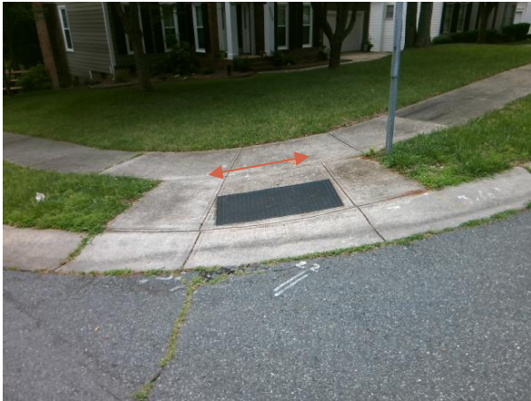
Curb Ramp Cross Slope
