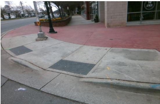
Curb Ramp Detectable Warning Surface
