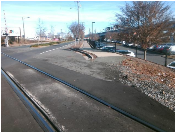
Missing Pedestrian Gate at Rail Crossing
