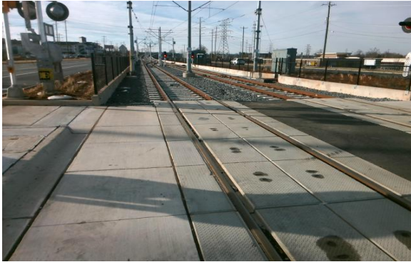
Rail Crossing – Missing Pedestrian DWS
