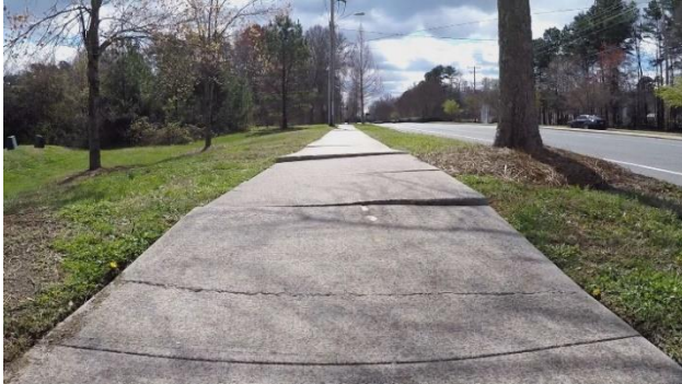
Sidewalk Obstruction – Uneven Heaving
