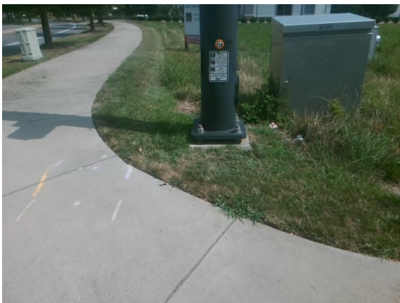
Pedestrian Signal – Pushbutton Side Reach
