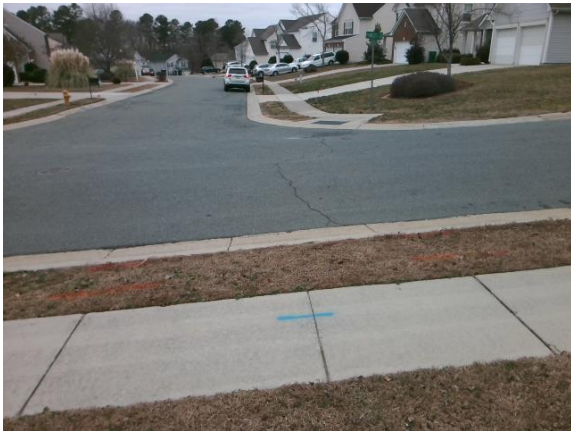
Missing Curb Ramp
