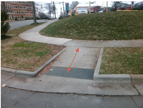
Curb Ramp Run Slope
