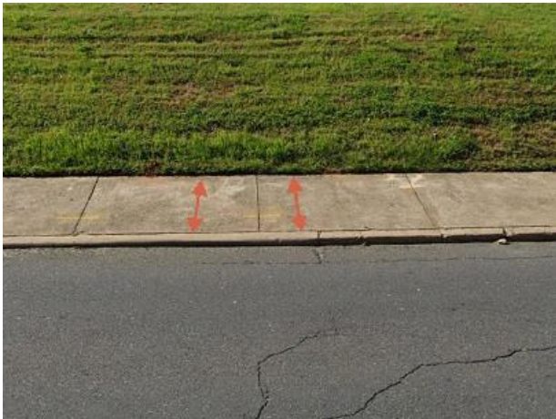
Sidewalk Cross Slope, as depicted by arrows
