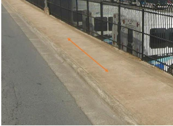
Sidewalk Run Slope, as depicted by the arrow
