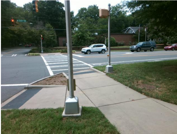
Pedestrian Signal – Clear Space Slope
