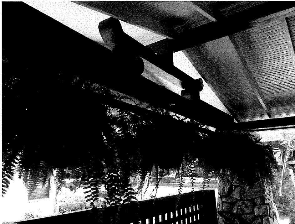
Side Porch Rafters
