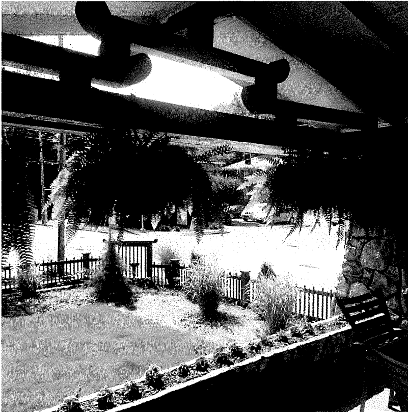
Front Porch Rafters
