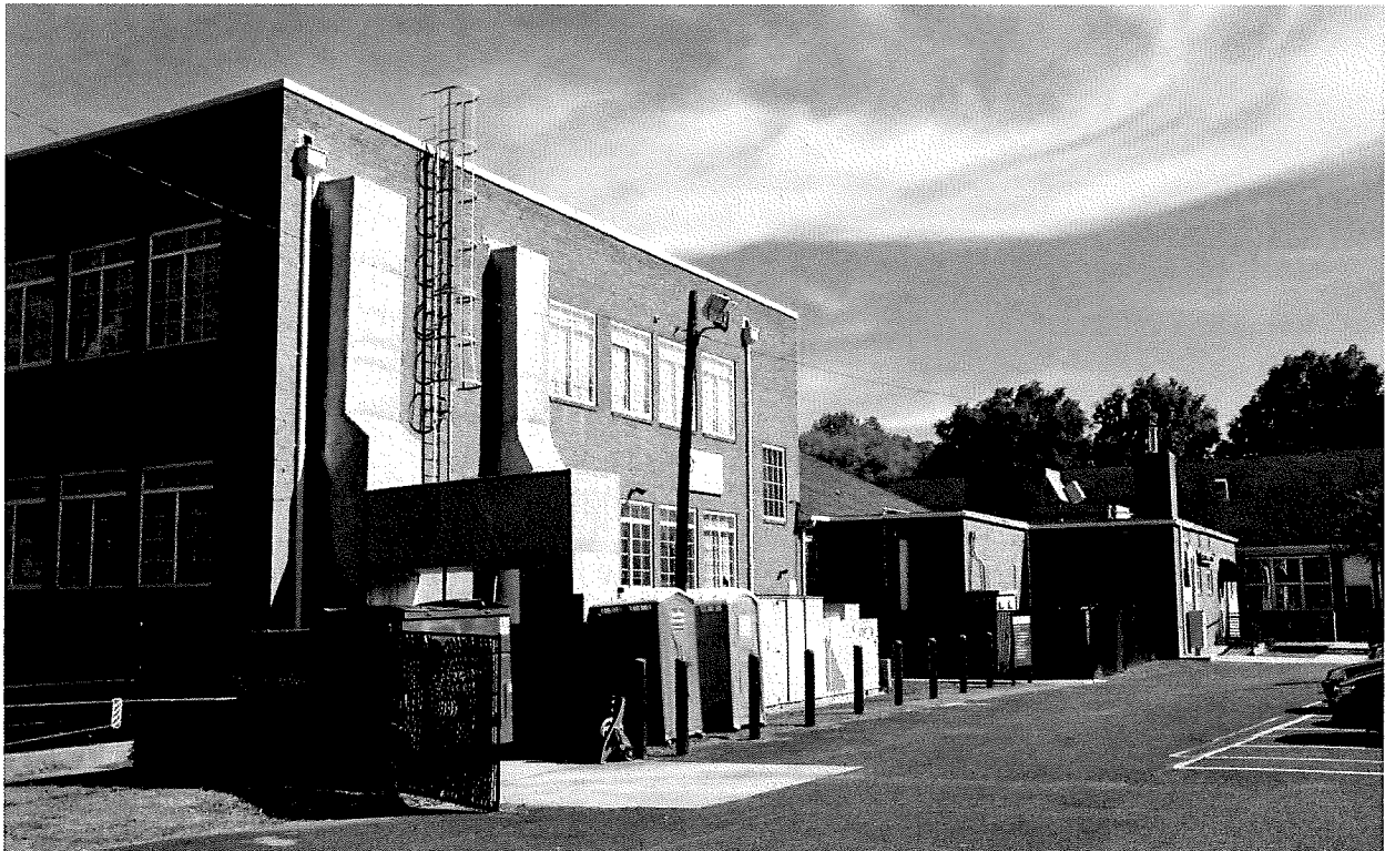
Figure 14 West elevation of the multi-level classroom building and the cafeteria expansion.
