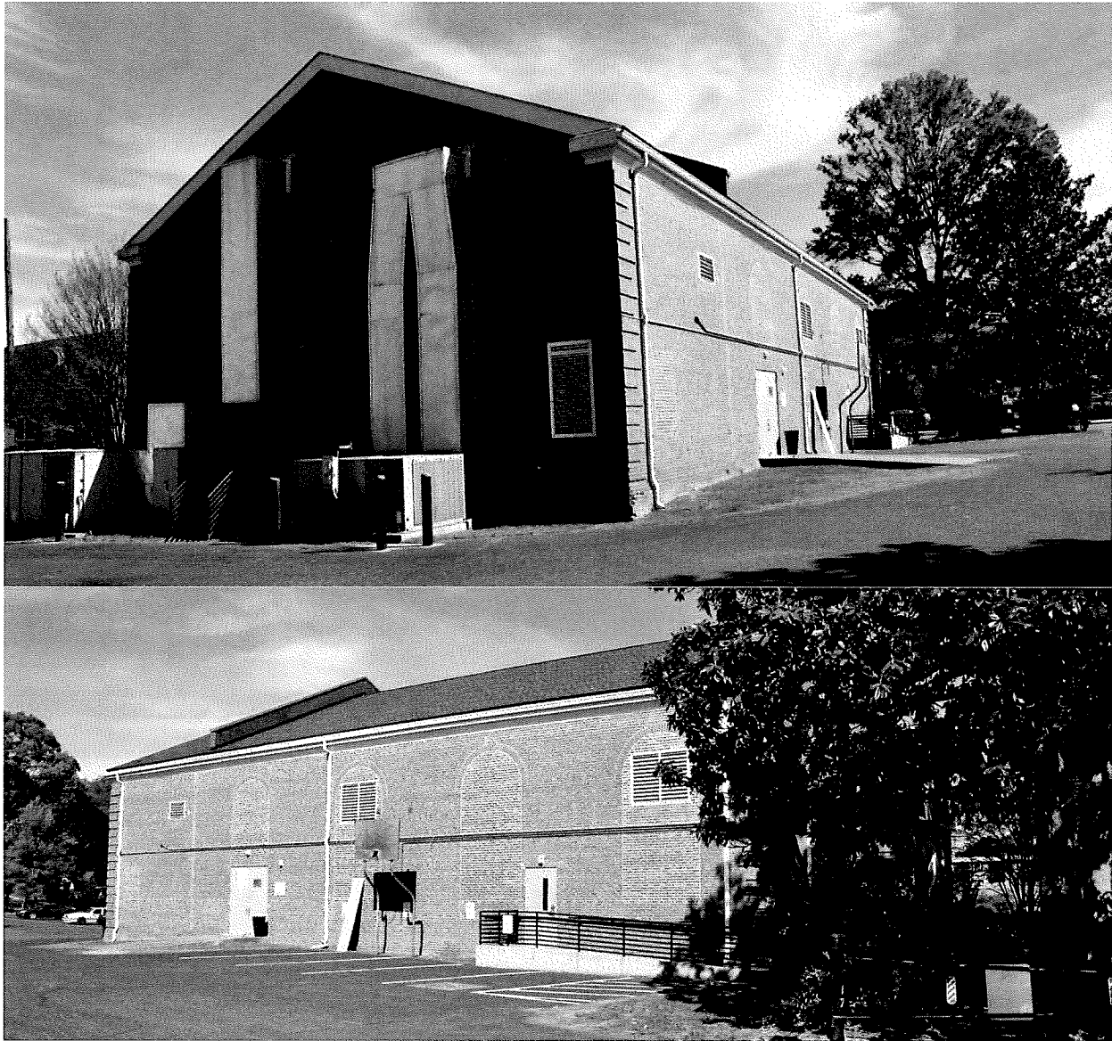
Figure 16 The north (top) and west (top and bottom) elevations of the auditorium/gymnasium.
