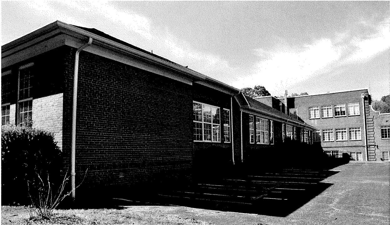
Figure 11 East elevation of the original building and the circa 1937 addition.
