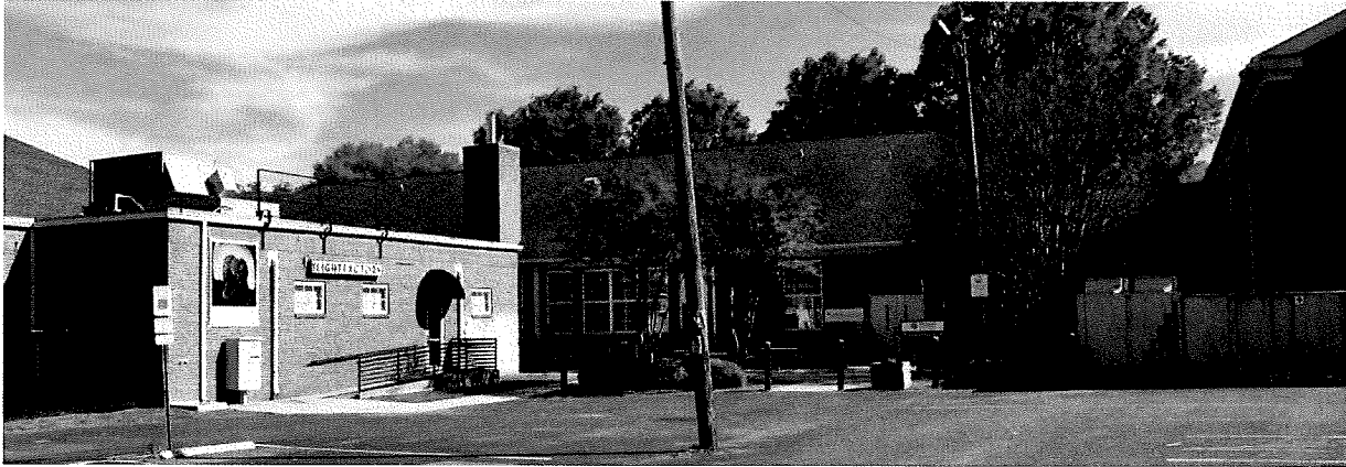
Figure 15 The north elevation of the original building.
