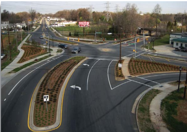
The intersection of Rozzelles Ferry and West Trade Street was retrofitted to improve safety for all travelers by removing a high-speed turn lane, providing dedicated turn lanes in all directions, and installing sidewalks, crosswalks, landscaped median islands, and bike lanes
