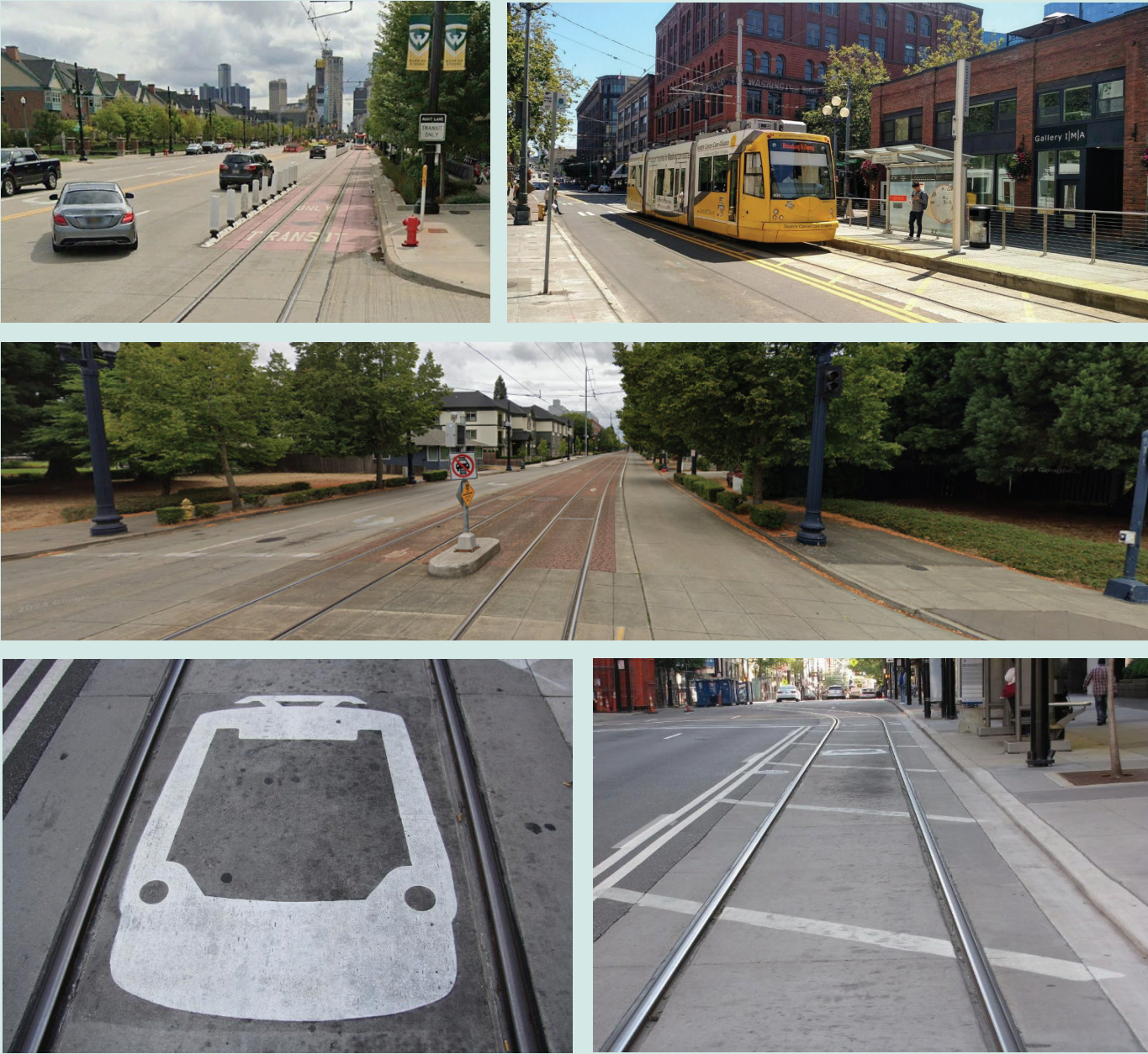
The images above illustrate dedicated guideway design treatments for other streetcar facilities in Detroit, MI; Seattle, WA; Hillsboro, OR; and Cincinnati, OH. The design team studied these precedents, and others, to understand the feasibility of establishing a dedicated guideway for the Gold Line streetcar through the West End interchange area.
