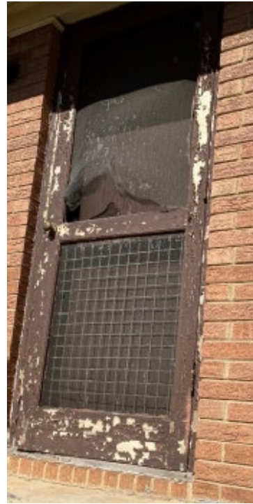
Side Door Change. All wood panel door with wood screen door.
