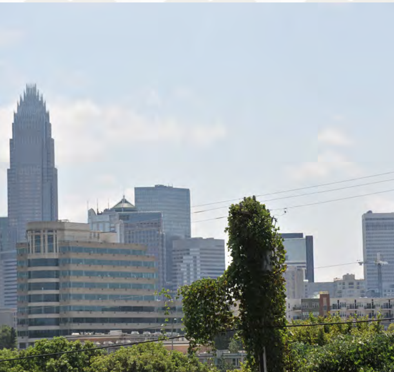
View of Uptown skyline from the Tarlton Hills Neighborhood
