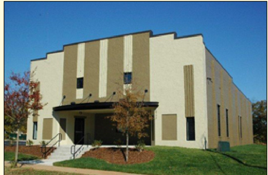
Pictured above is the front of the new Belvedere Theatre as it neared its opening day at Charlotte. Equipment was furnished by National Theatre Supply while the Hubert Mitchell Industries of Hartsville, Ala., installed the curtains and draperies. In the adjacent photo are Arthur and Herbert Sherman, owners of the new theatre.
