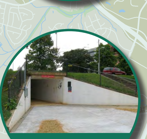
Charlottetown Dr Ped/Bike Tunnel
