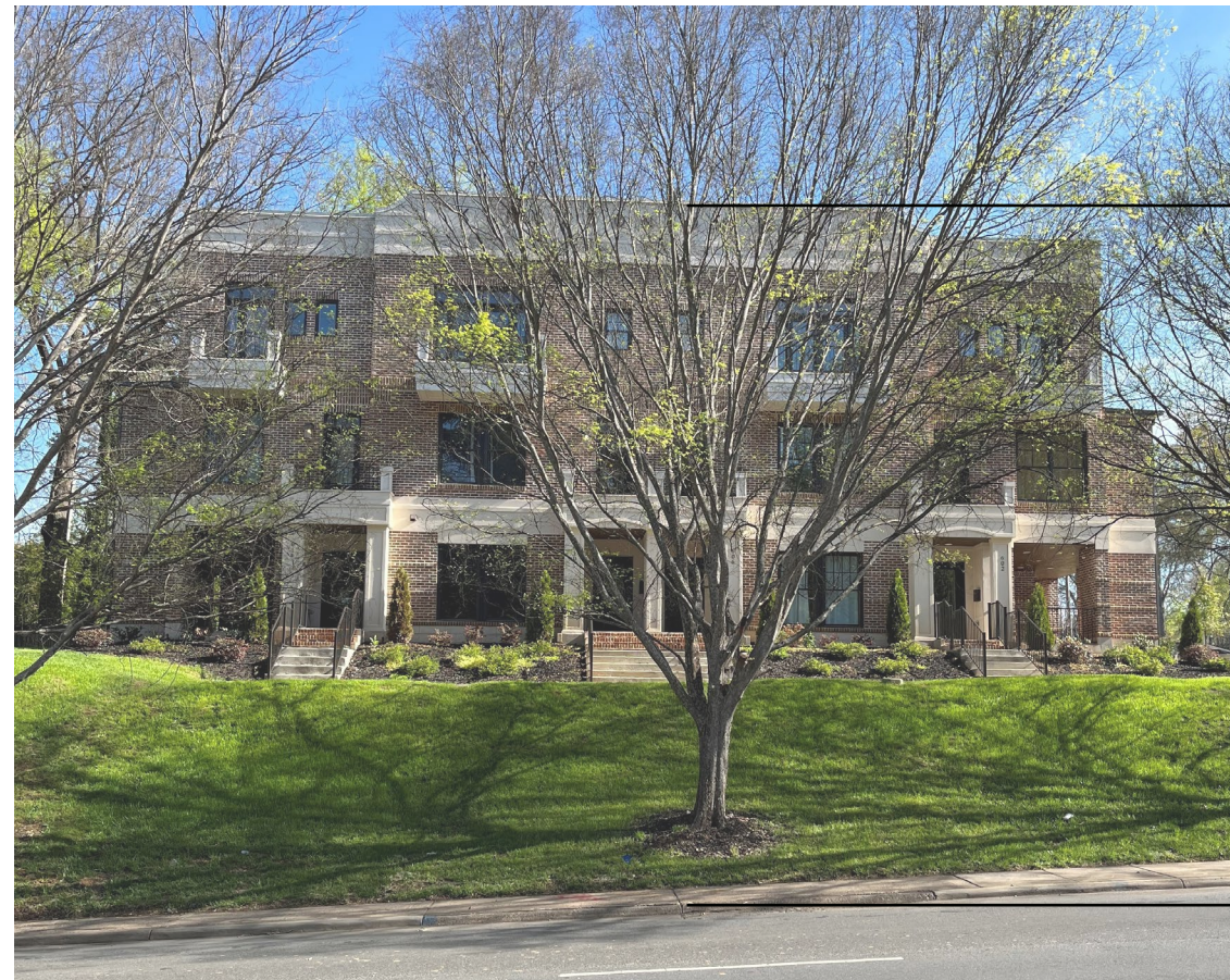
Worthington and West Townhomes - 600ft from site
