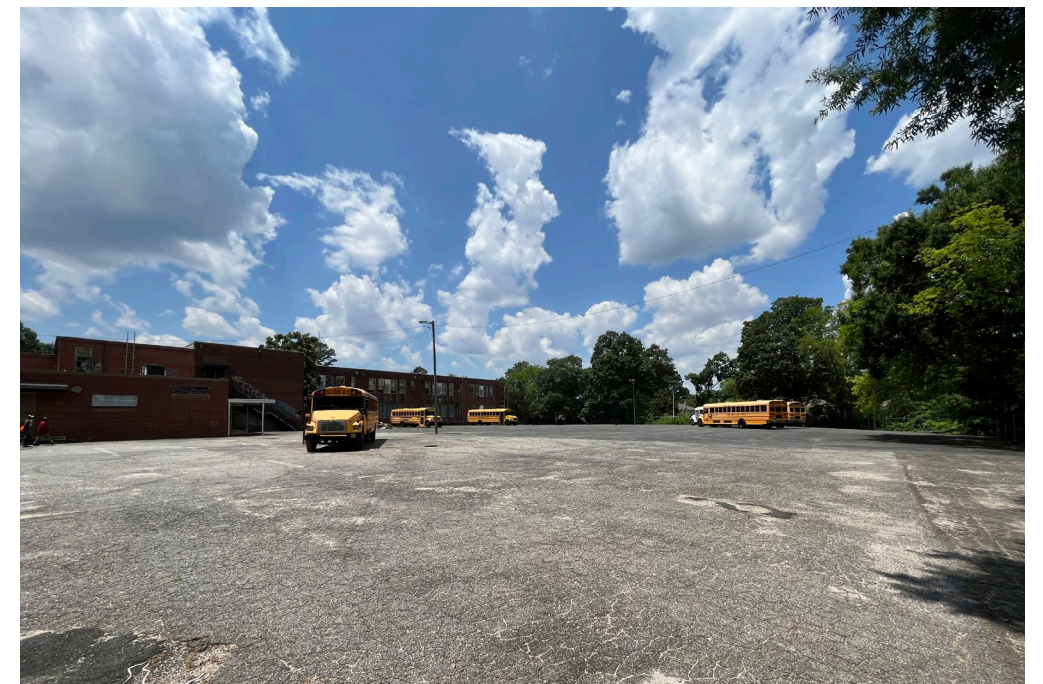
Rear Parking lot View, Wilmore School
