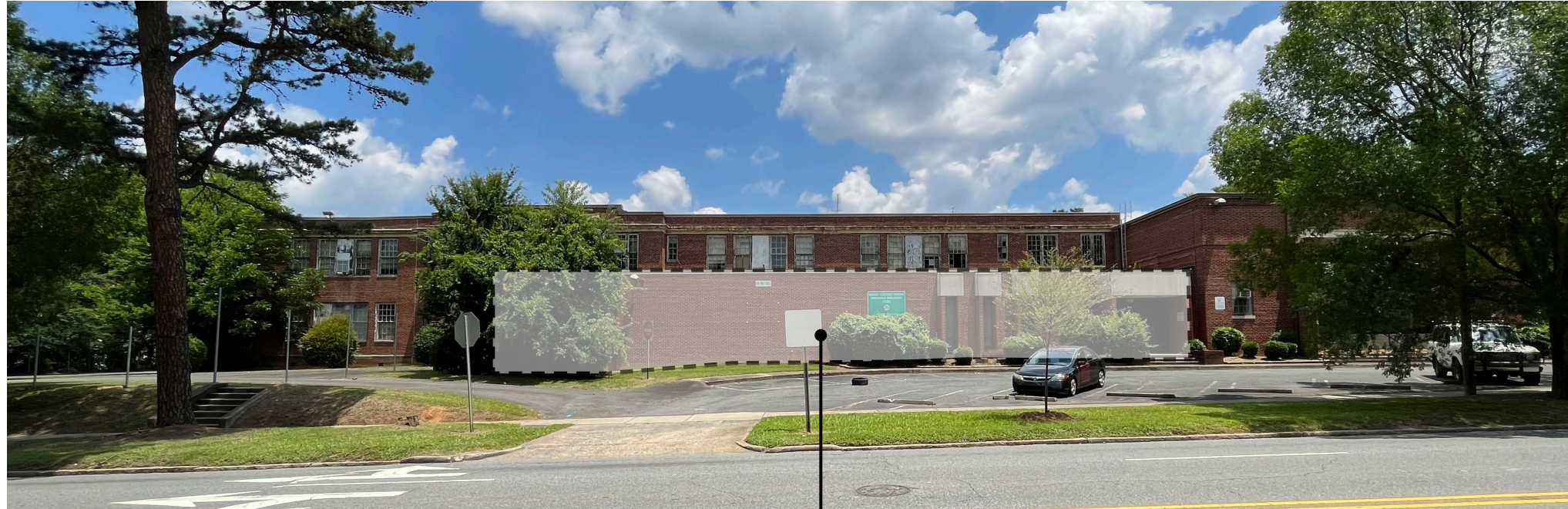
West Blvd, Front elevation of Wilmore School
