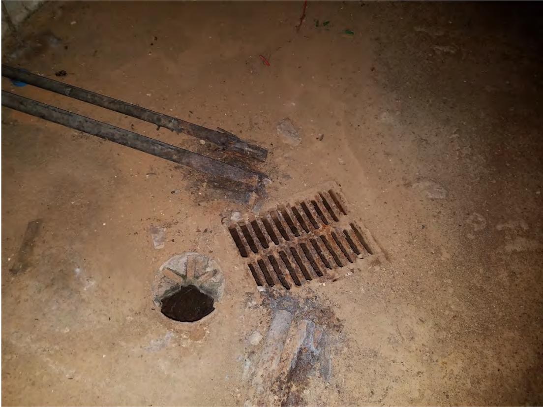
Photograph 13: Floor drain located in the boiler room
