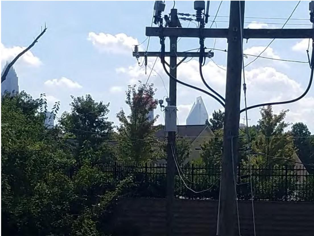
Photograph 15: Pole-mounted transformer located adjacent to the southern Site boundary
