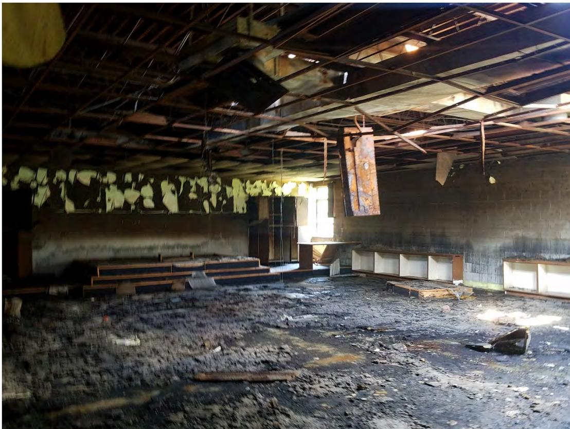
Photograph 12: Fire damage in the central portion of the Site building
