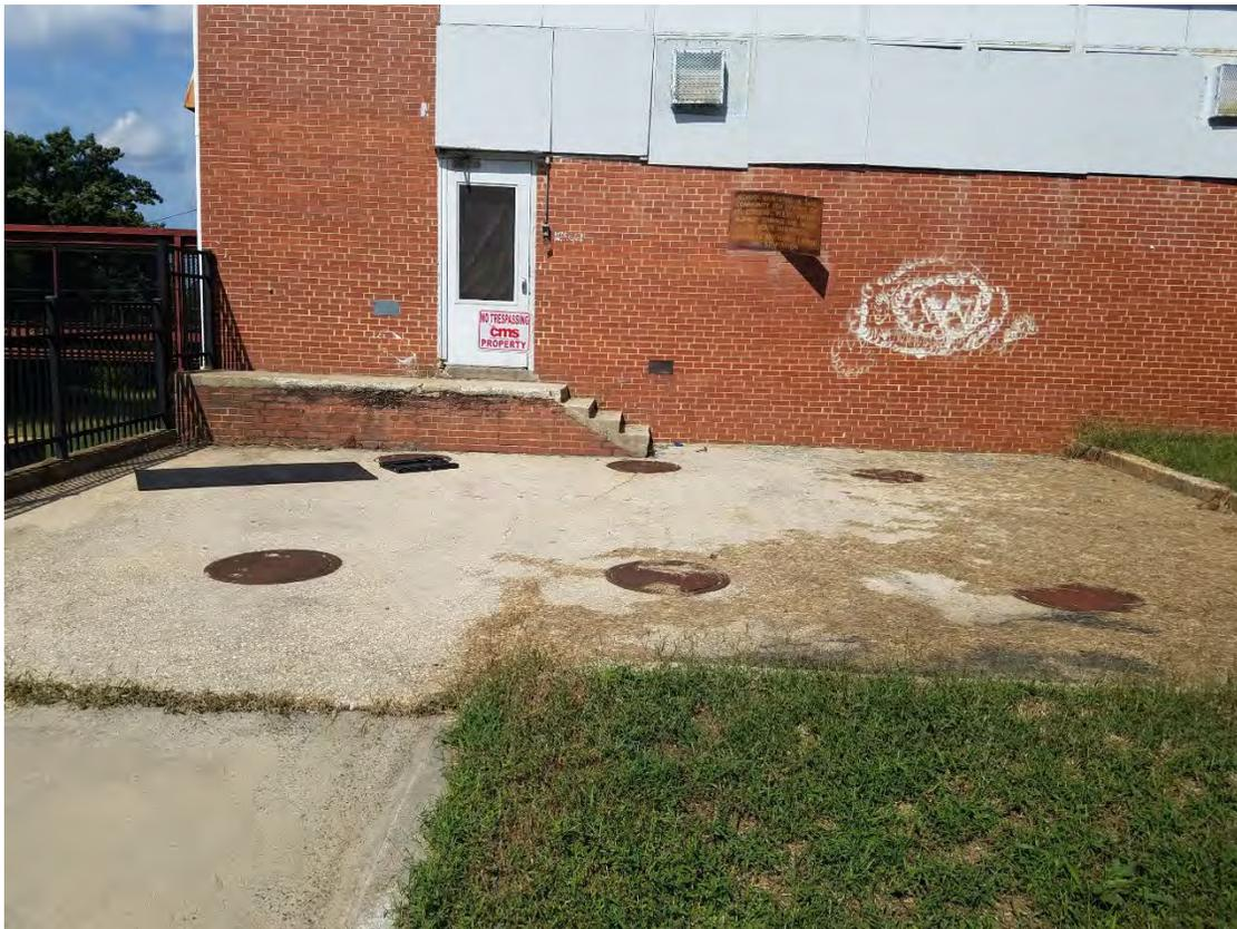
Photograph 10: Manhole covers located above a suspected coal vault in the boiler room
