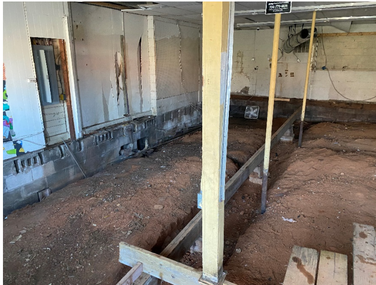
Picture 8 – Crawl Space with Removed Floor
