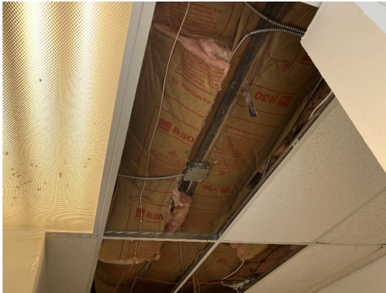
Picture #10 – Roof Structure
