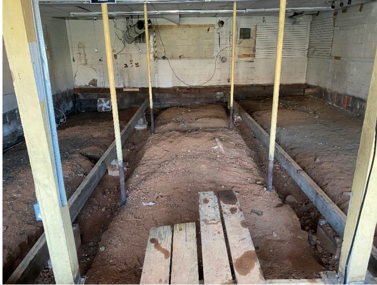
Picture #9 – Crawl Space with Removed Floor
