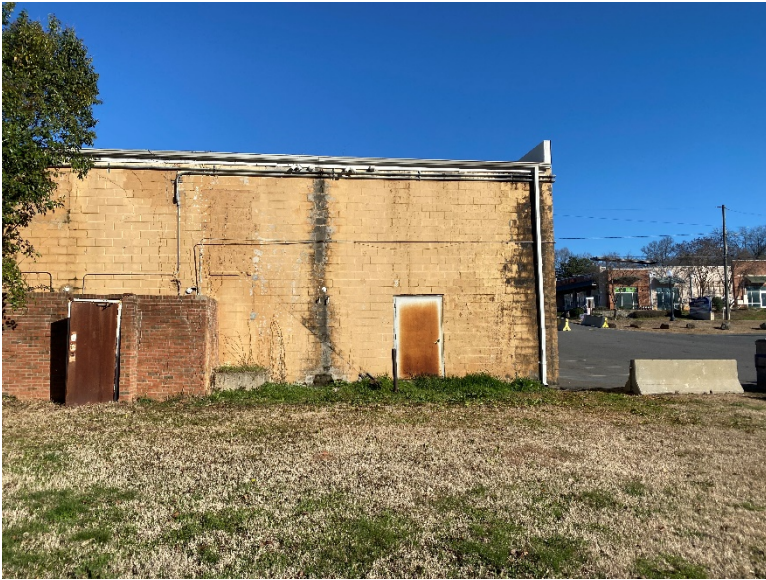
Picture #1 – Rear Exterior Wall
