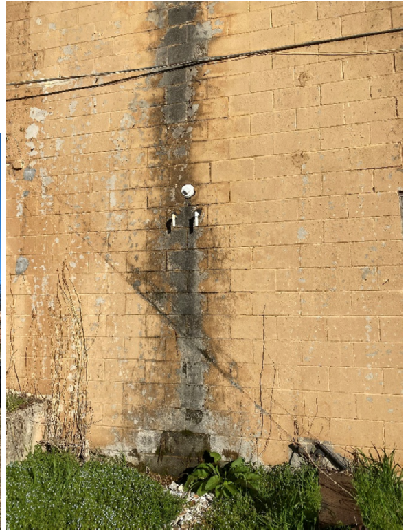
Picture #2 – Eastern Exterior Wall
