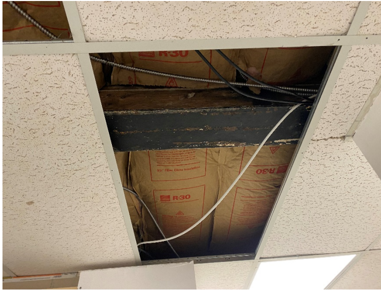
Picture #11 – Roof Beam Supporting Roof Joists
