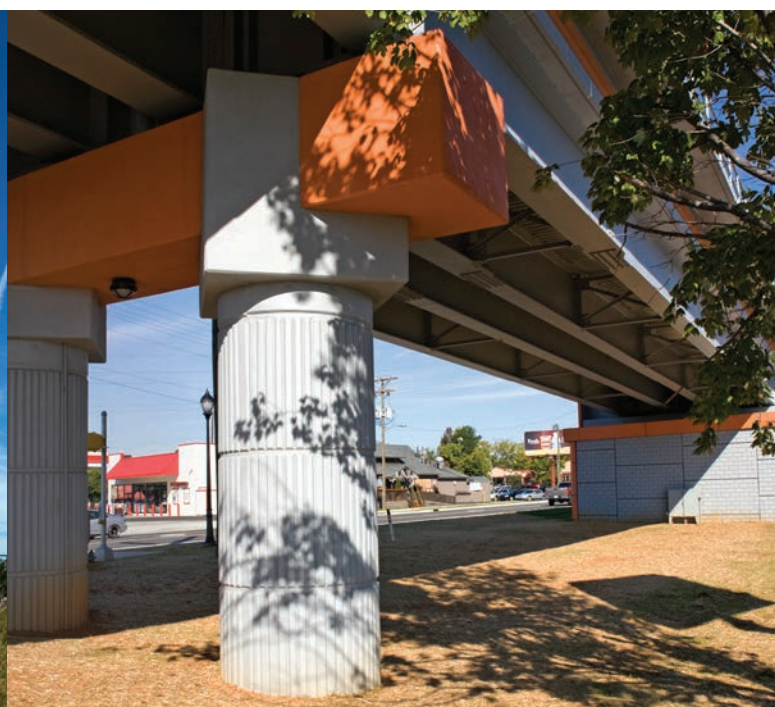
Woodlawn Marek Ranis, Bridge & Wall Enhancements
