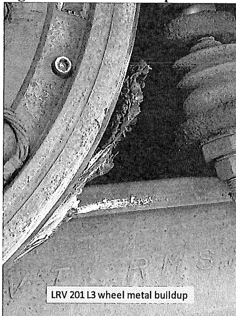
Figure 6 – Metal Buildup on Derailed Wheel
