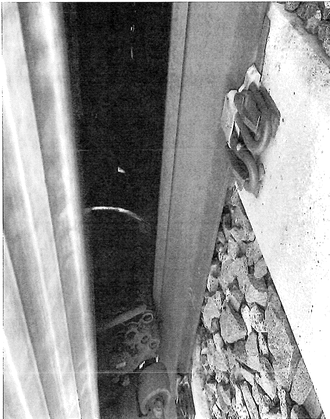
Figure 5 Center Truck Derailment
