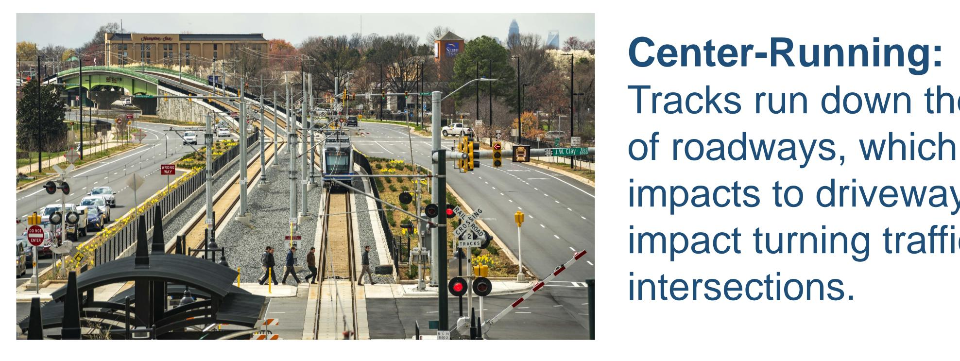
Tracks run down the middle of roadways, which reduces impacts to driveways but may impact turning traffic at intersections.
