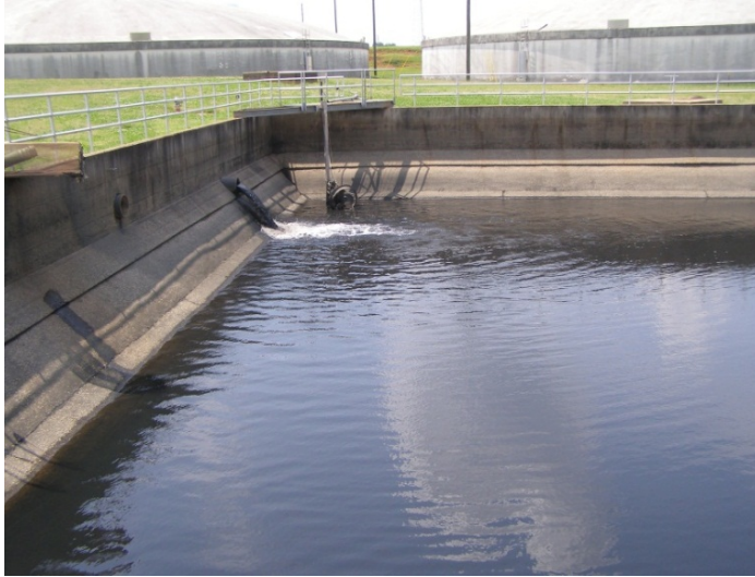
Figure 2-3 Spent Backwash Water Lagoon at Franklin WTP
