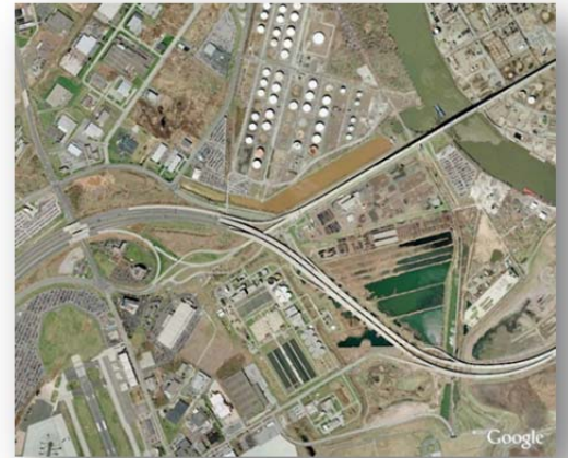
PWD Biosolids Recycling Facility
