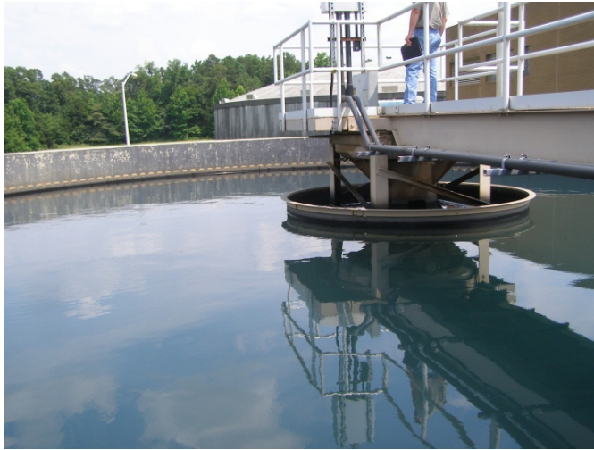
Figure 2-4 Gravity Thickeners
