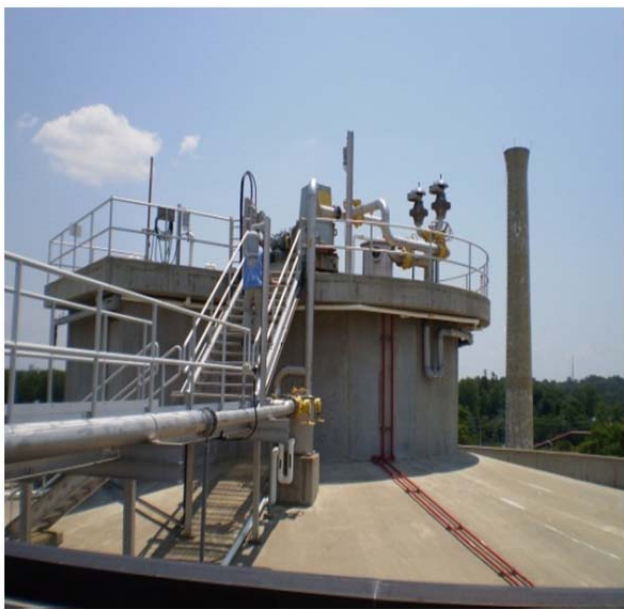
Figure 4-4 Anaerobic Digester
