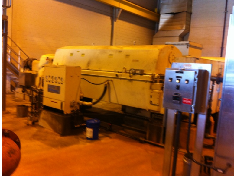
Figure 4-6 Dewatering Centrifuge
