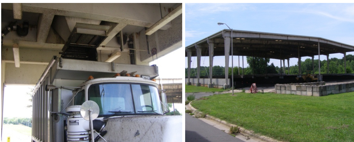
Figure 4-18 Solids Hauling and Storage
