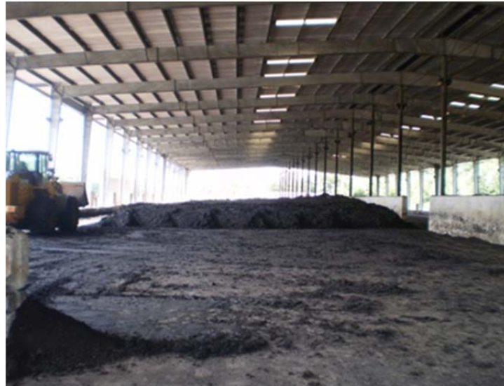
Figure 4-10 Covered Biosolids Storage Area
