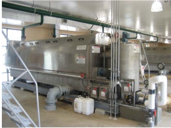
Figure 8-2 Rotary Drum Thickening
