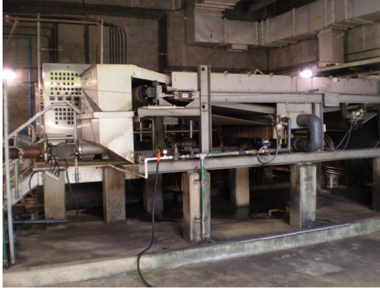
Figure 4-8 Gravity Belt Thickener
