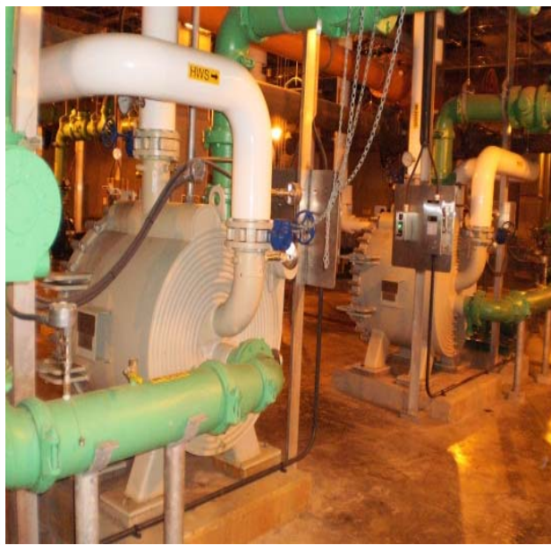
Figure 4-5 Heat Exchanges in Digester Complex
