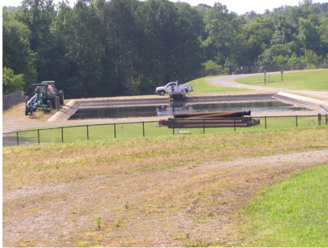
Figure 2-12 Lee S. Dukes WTP Thickened Residuals Storage Lagoon
